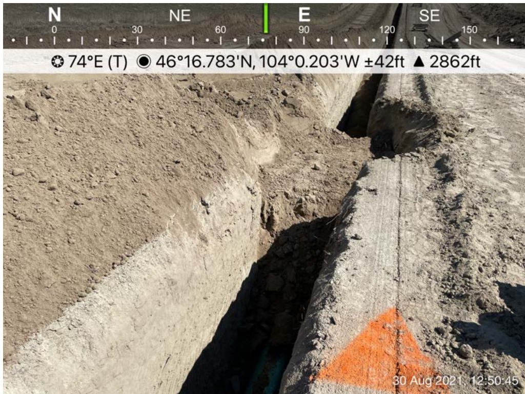
Photo #2 "Pipe Lowered and being Backfilled with Subsoil"
