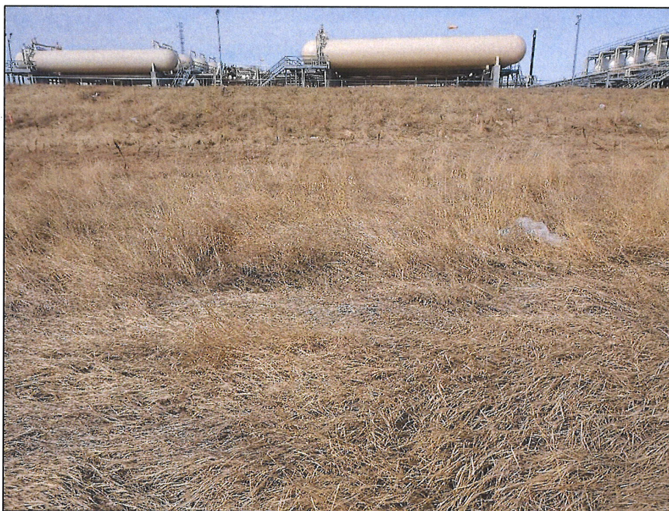
Additional survey area near MP 12 facing W
