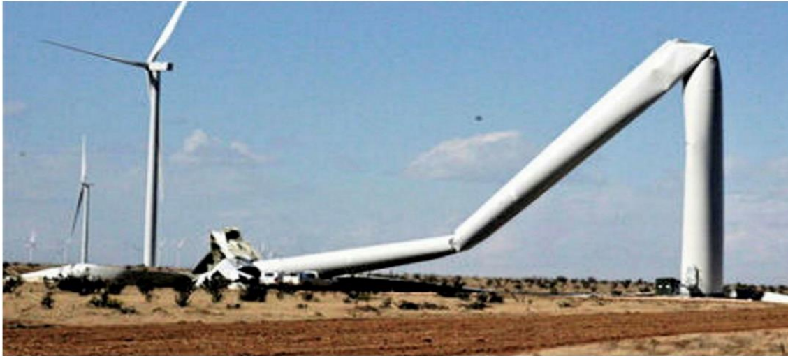
Toppled turbine at NextEra Energy Resources' Casa Mesa Wind Energy Center in New Mexico Photo: Shawna Shoemaker Stowe via Facebook
