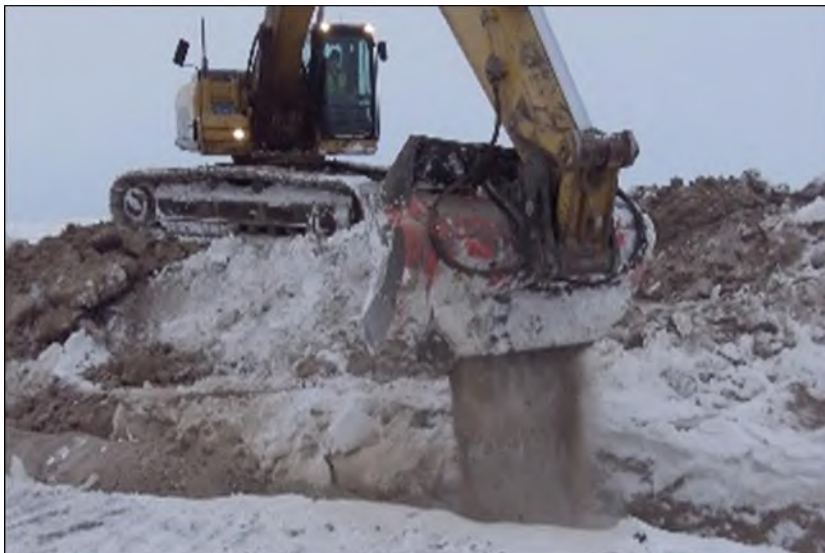
Shaker Equipment Backfilling Trench
