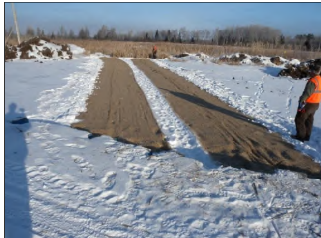
Stabilization of the Right-of-Way
