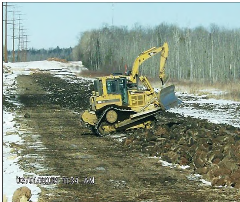
Reducing Frozen Crown Over Backfilled Trench
