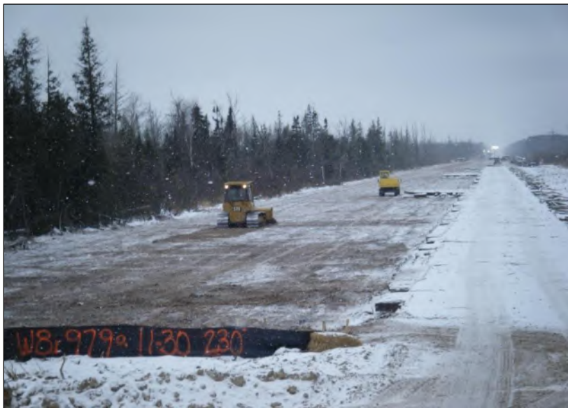
Preparing the Right-of-Way
