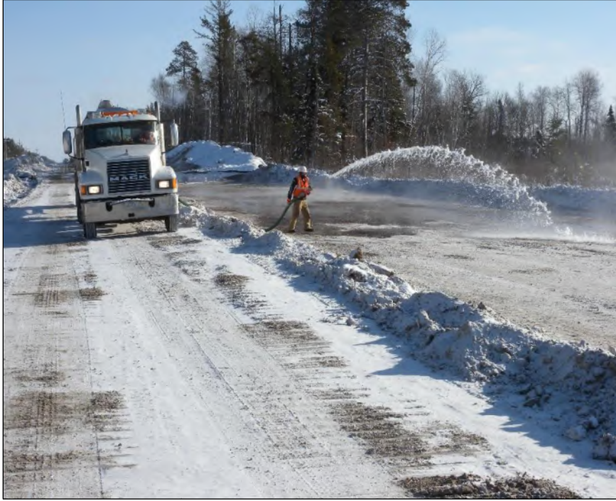
Building the Ice Road
