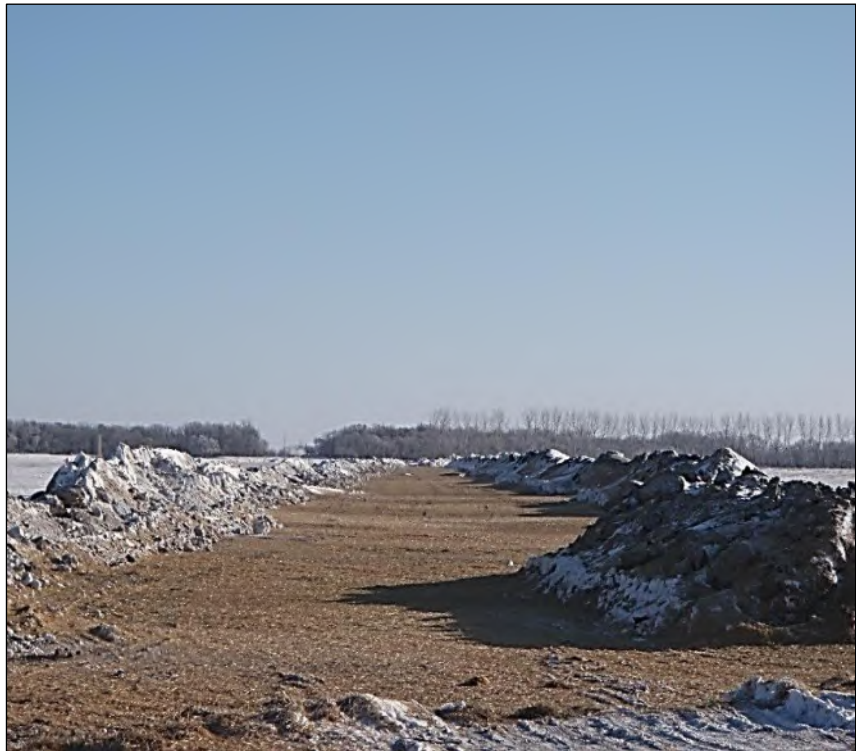
Right-of-Way Prepared for Final Stabilization
