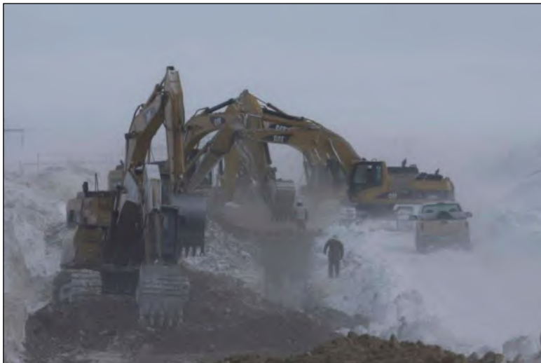
Pipeline Construction in Frozen Conditions
