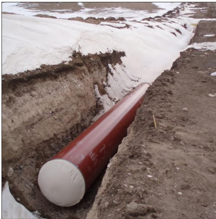
Pipeline Construction in Frozen Conditions
