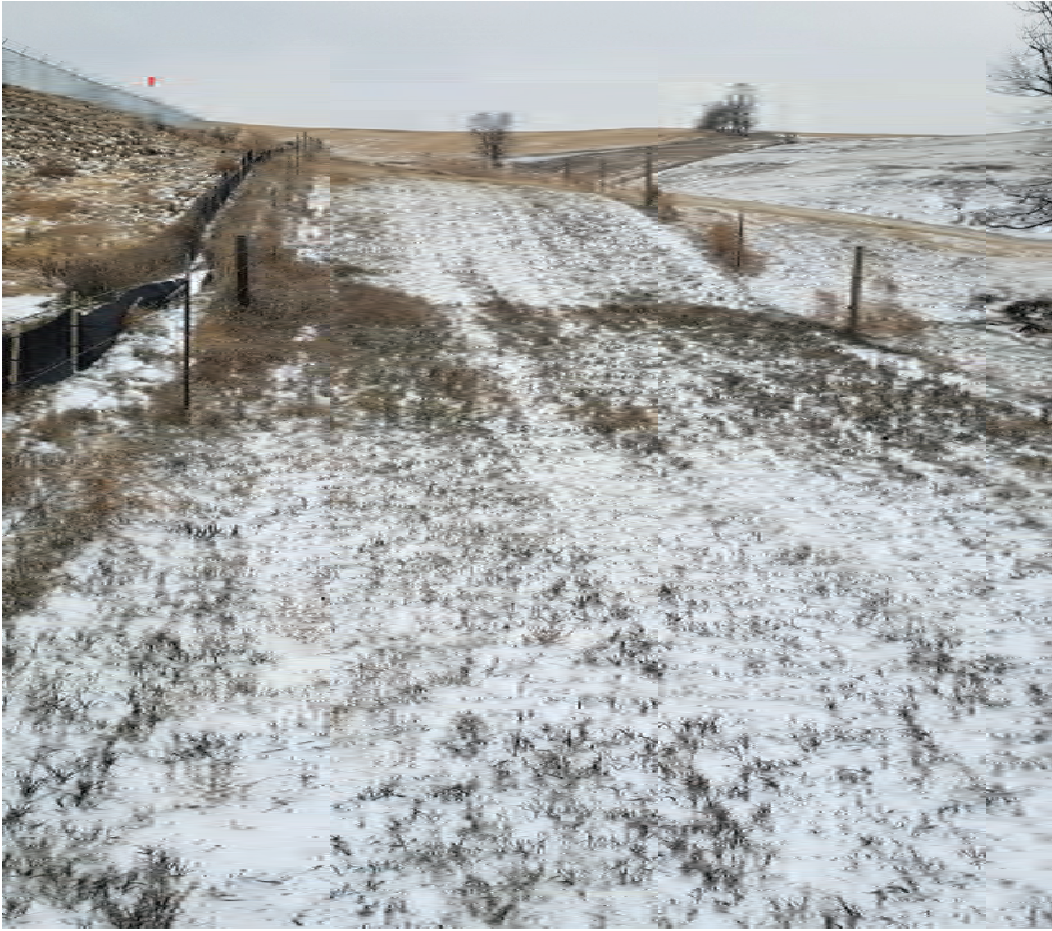
P7 – West Boundary facing South at Site Low Point Drainage Exit
