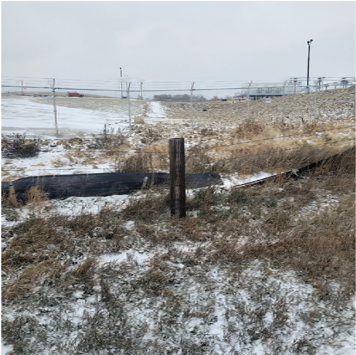
P23 – Low Point Site Drainage Exit Facing East
