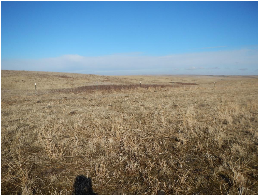
Photo 39. WTL-009 drainage from pipeline crossing, facing west/northwest. Picture taken on March 26th, 2020.
