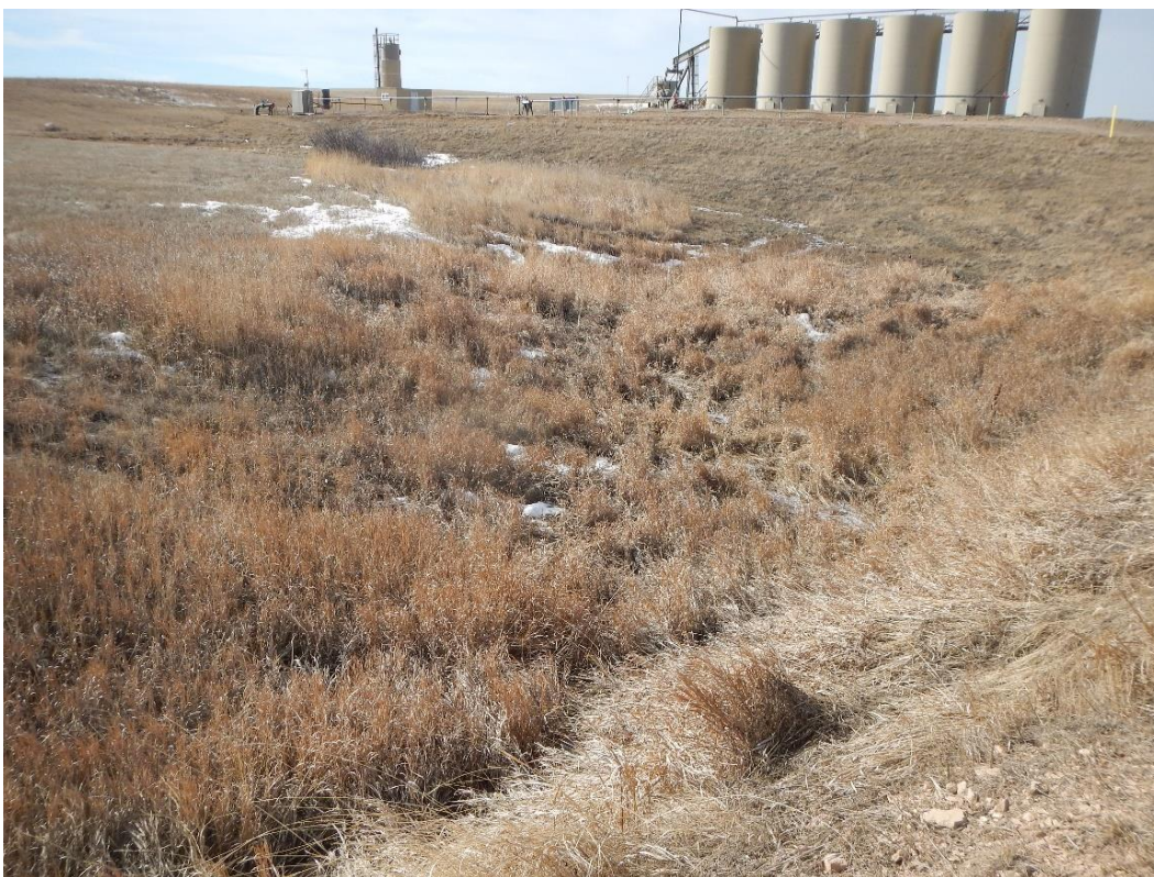
Photo 4. WTL-001 drainage upstream of crossing and existing road, facing south. Picture taken on March 6th, 2020.
