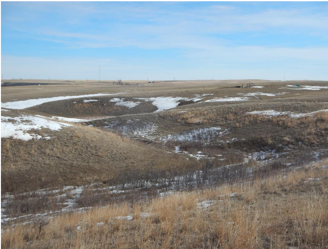
Photo 3. WTL-001 drainage downstream of crossing, facing northeast. Picture taken on March 6th, 2020.
