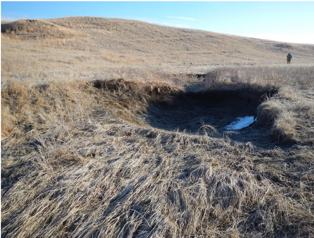
Photo 31. WTL-006 drainage downstream from crossing, facing northeast. Picture taken on March 26th, 2020.
