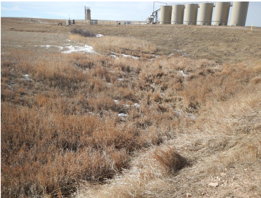
Photo 4. WTL-001 drainage upstream of crossing and existing road, facing south. Picture taken on March 6th, 2020.
