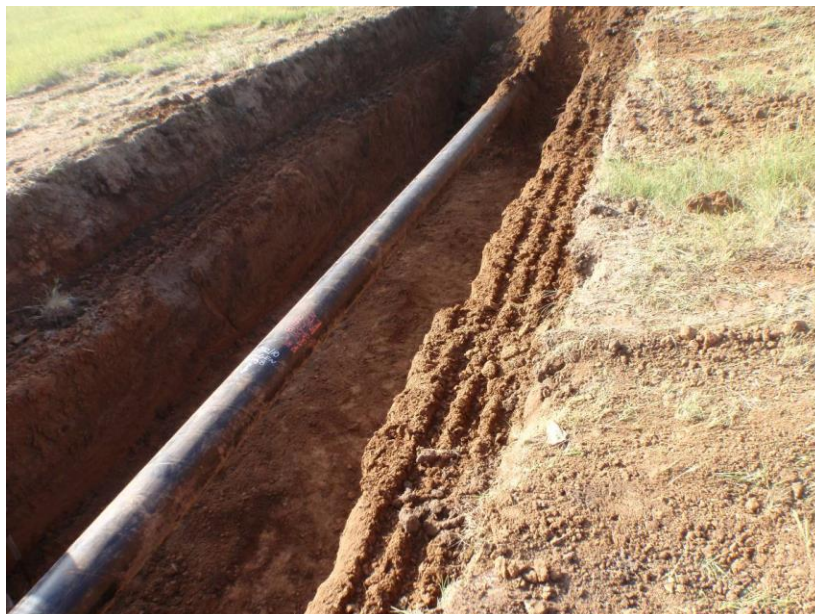
Figure K-2. Example Excavation Condition Photograph
