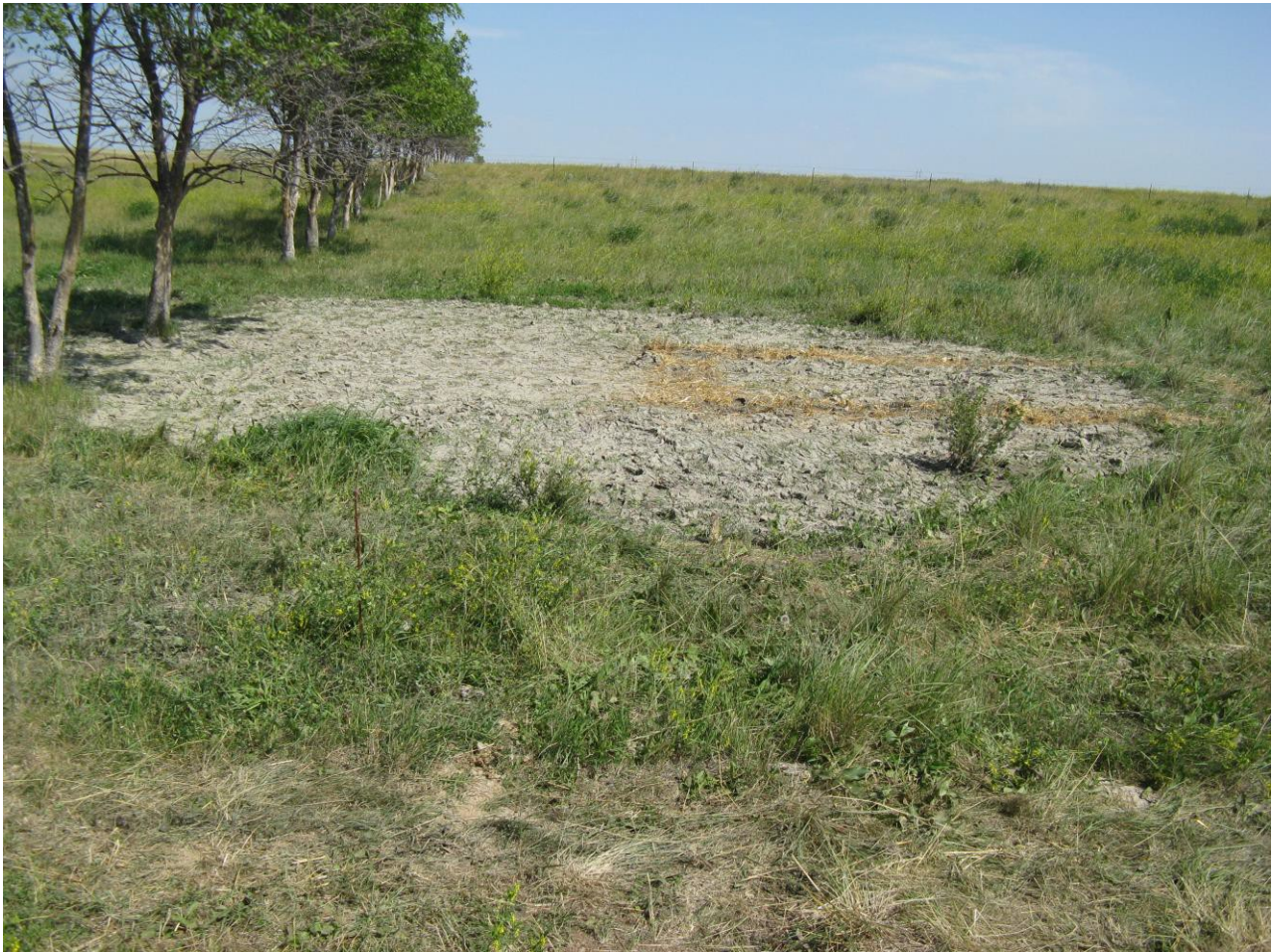
Figure 2. Typical Surface Expression of a Frac-Out
