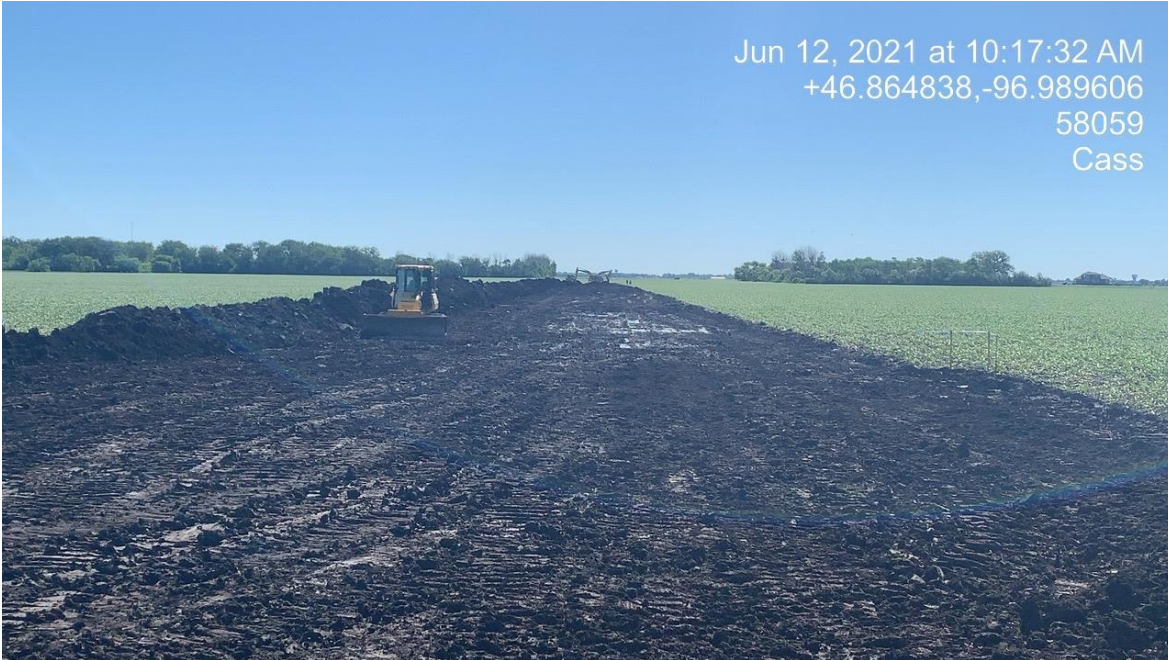
Top soiling operations started.
