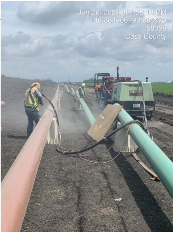
Sandblasting and preparation fo pipe field joints for coating
