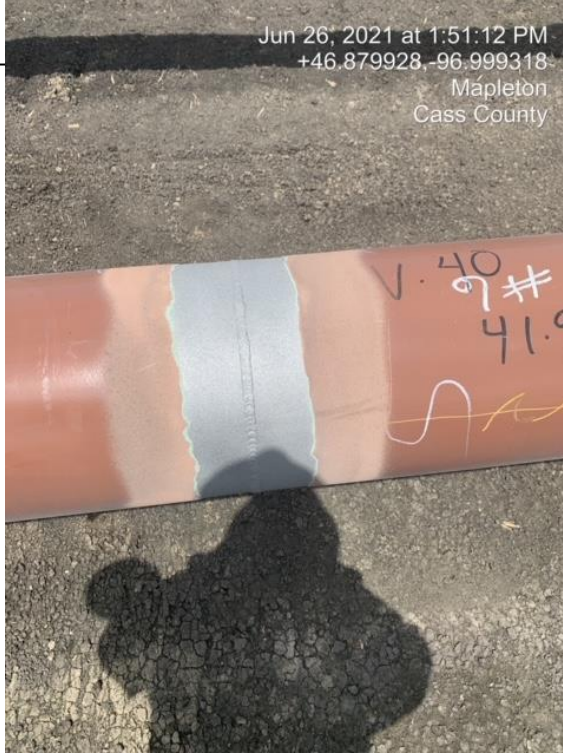
Sandblasting and preparation fo pipe field joints for coating
