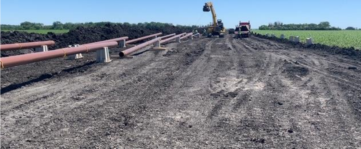
Pipe stringing along right-of-way
