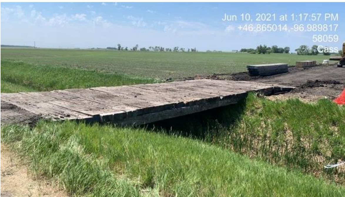
Bridging installed at 166 th Road and over wetland for field access.
