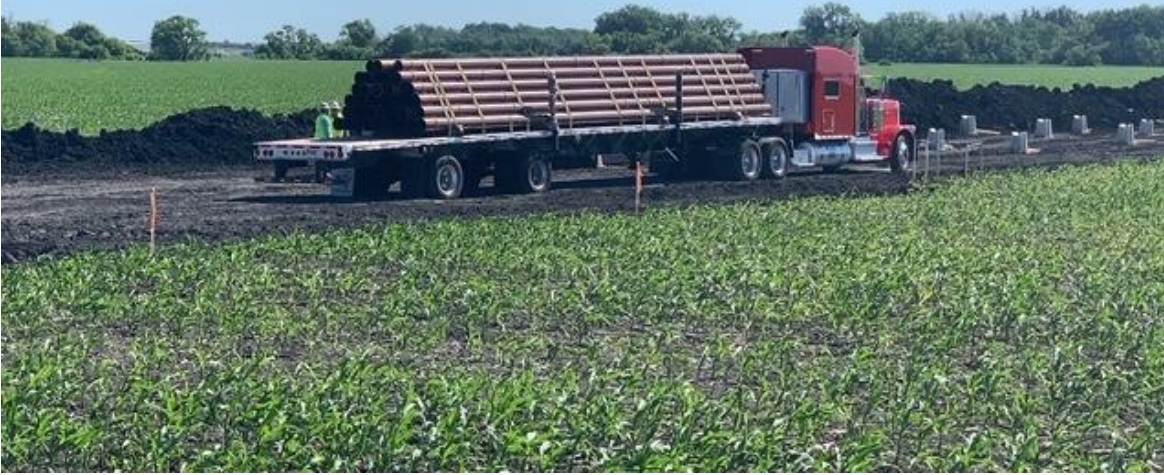
First loads of pipe being delivered to site
