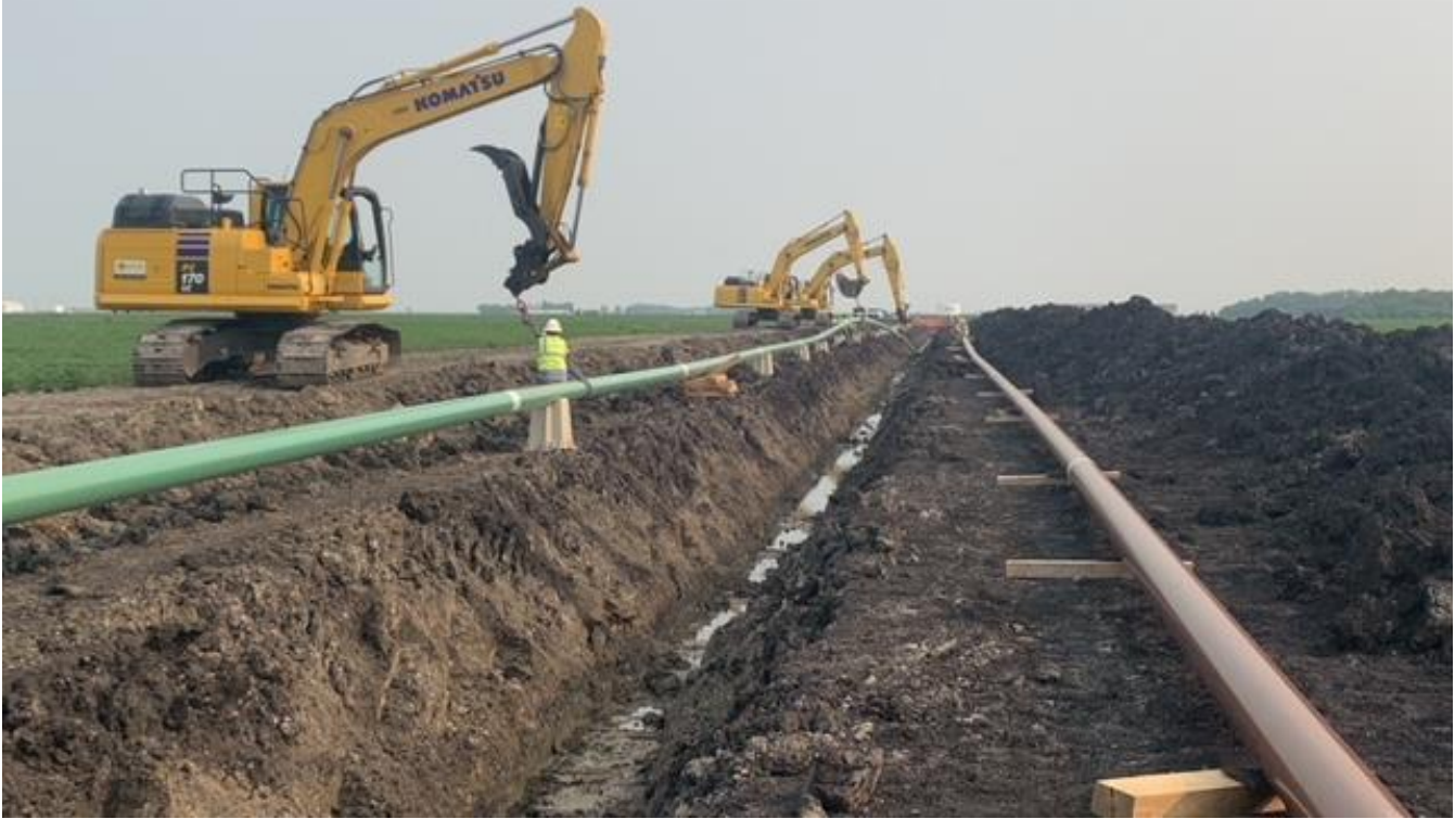
Laying in of mainline section of pipe
