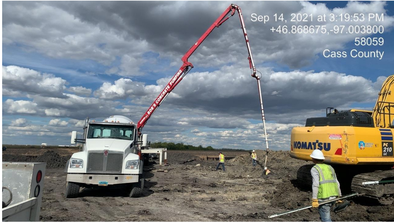
Grouting operations for Drain 14 HDD cavity
