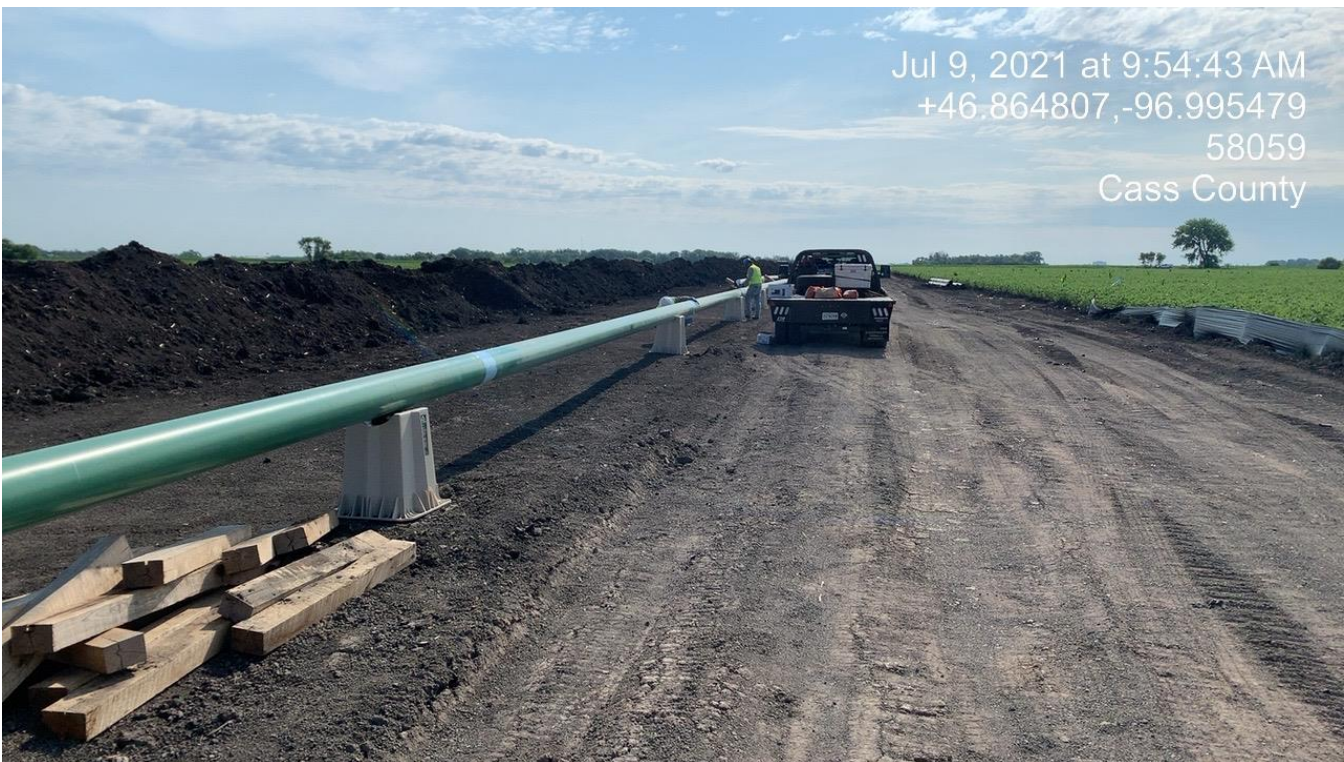
Pipe joint coating applications
