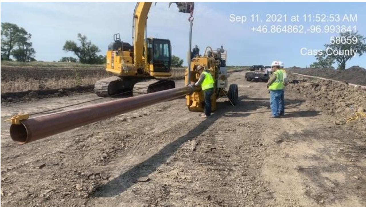
Pipe bending activity.
