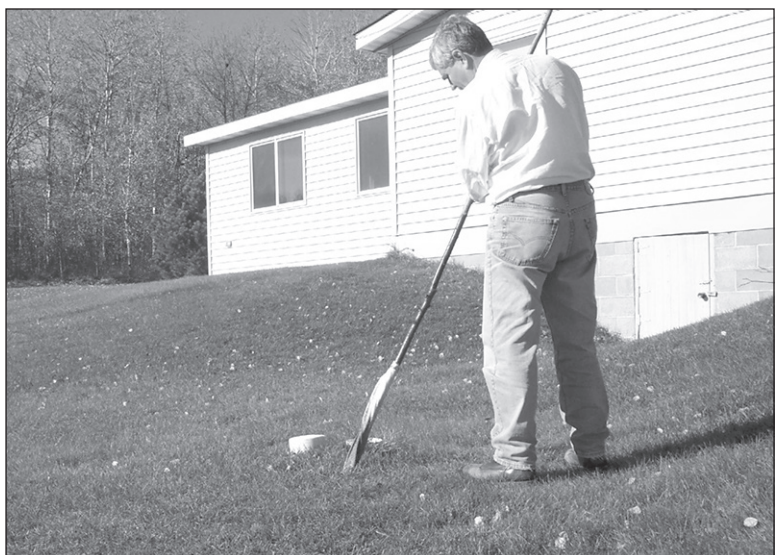
Tom Scherer, NDSU Extension agricultural engineer, shows how to measure the depth of sludge in a septic tank.
