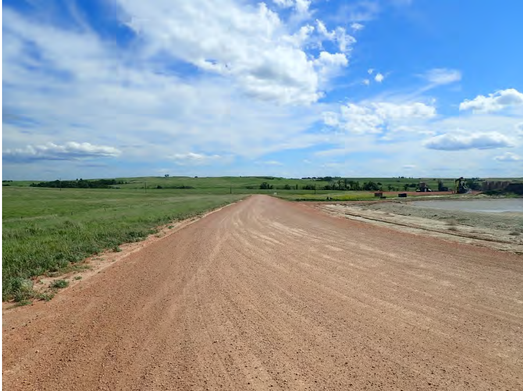
Figure 4. Overview photo of the survey area. View is to the south. (Photo was taken on July 14, 2020, by Alex Atkinson. The image has not been altered.)
