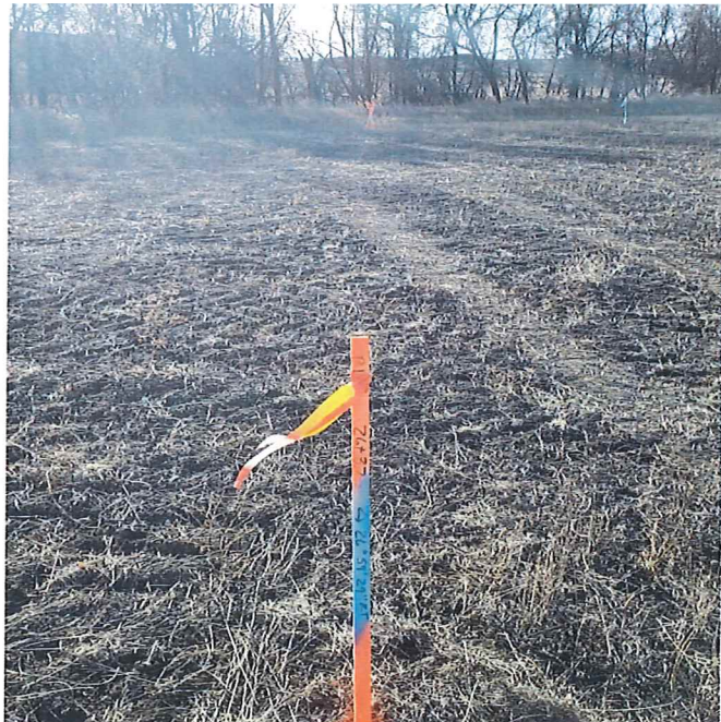
P8 - STA 26+37 AH, Existing Conditions
