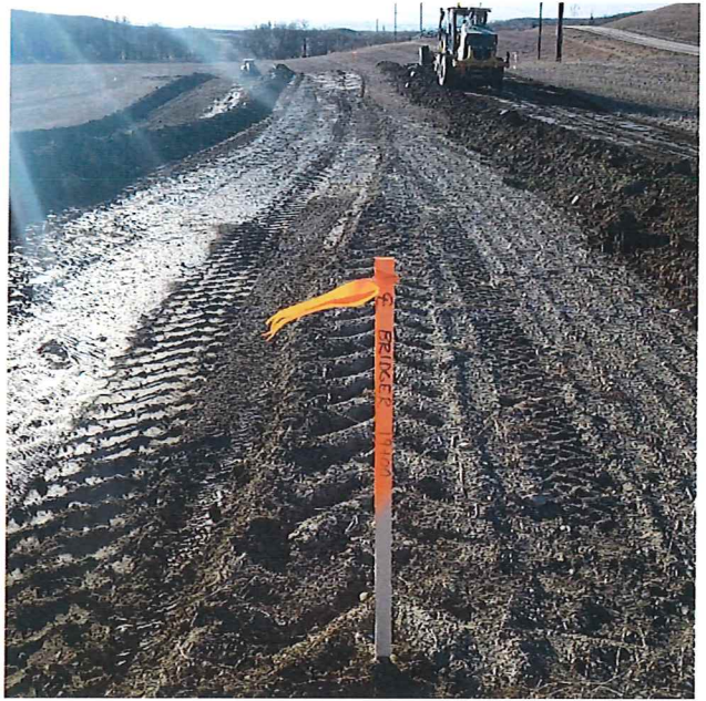
P36 - STA 19+00 AH, Topsoil Removal
