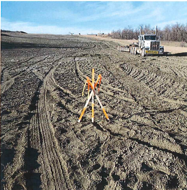
P18 - STA 58+18 AH, Existing Conditions, End Bore
