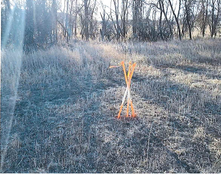
P9 - STA 27+38 AH, Existing Conditions, Bore Begin
