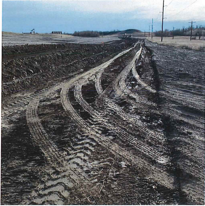
P40 - STA 38+50 AH, Topsoil Removal
