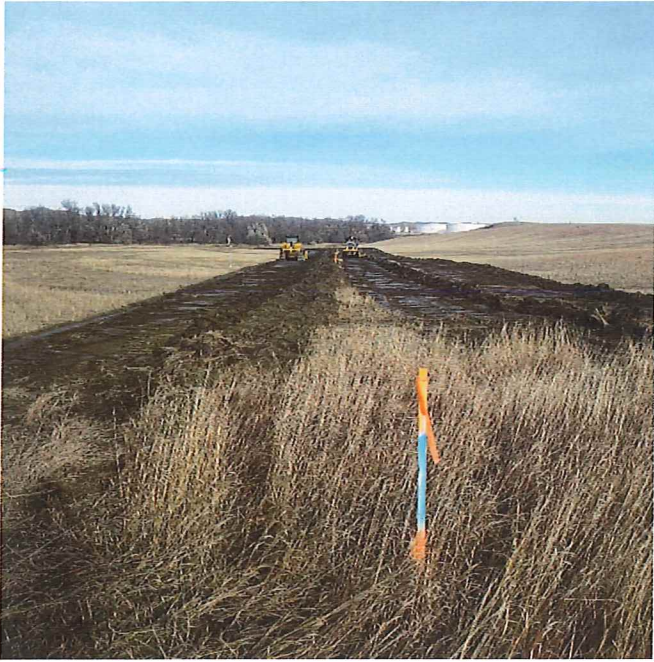
P39 - STA 37+82 BK, Topsoil Removal and Windrow
