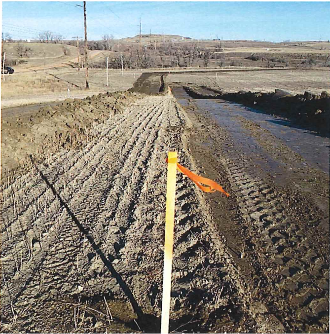
P37 - STA 19+00 BK, Topsoil Removal
