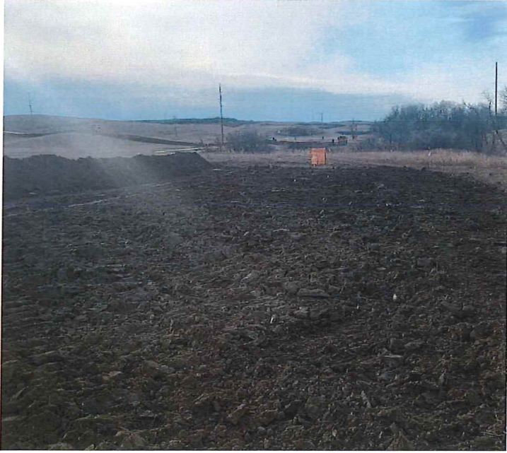
P35 - STA 8+00 AH, Topsoil Removal and Windrow
