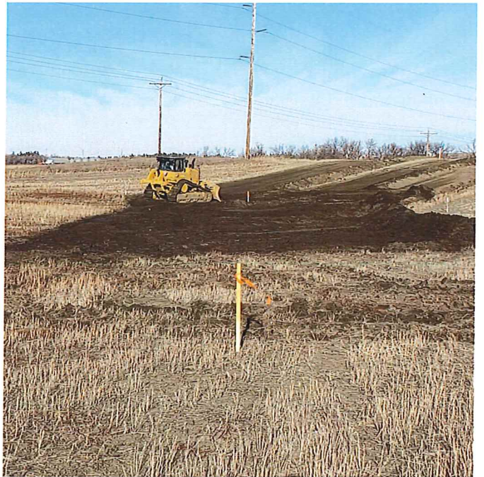
P38 - STA 24+00 BK, Topsoil Removal and Windrow
