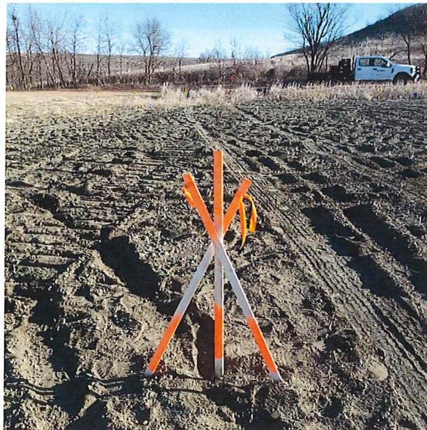
P19 - STA 58+18 BK, Existing Conditions, End Bore
