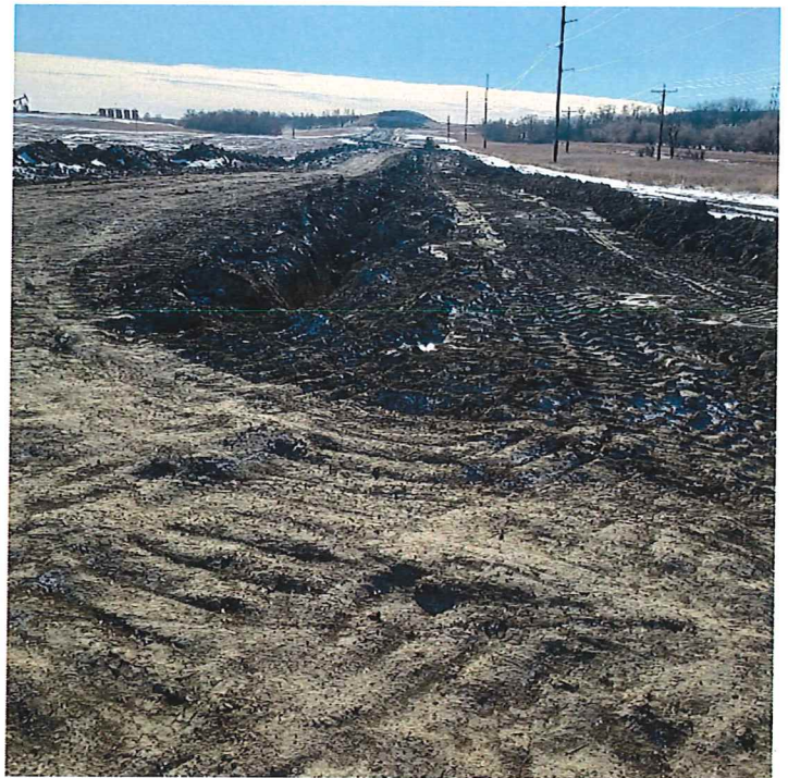
P33 – STA 38+50 AH_Trench Backfill
