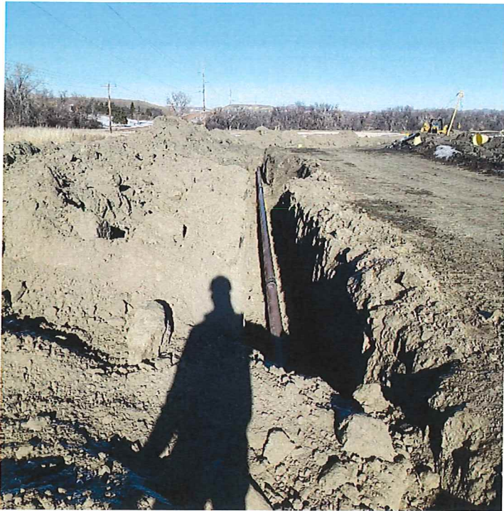
P32 – STA 38+50 BK_Trench
