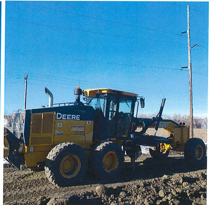
P45 – Equipment Onsite
