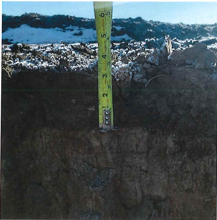
P16 – STA 15+42 Topsoil Remaining
