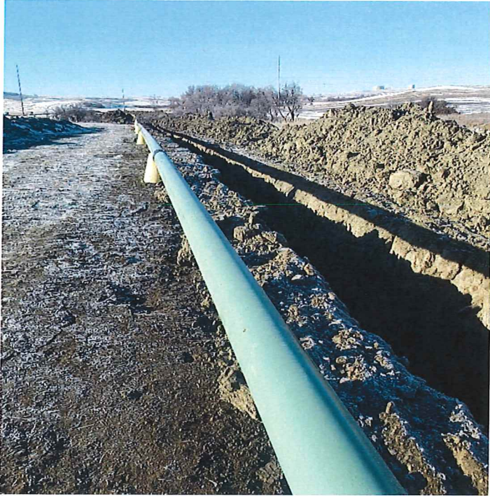
P4 – STA 8+00 AH_Welded 8 IN Pipe
