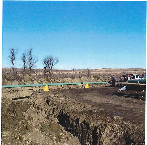
P41 – STA 14+50 BK_Pipe Welding
