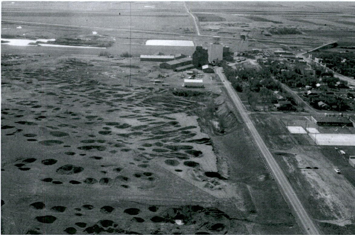
Photo 1: Sinkholes near Scranton, ND, circa 1980
