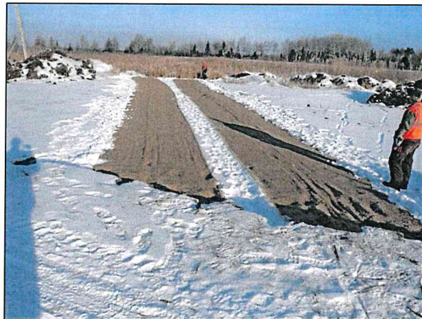
Stabilization of the Right-of-Way
