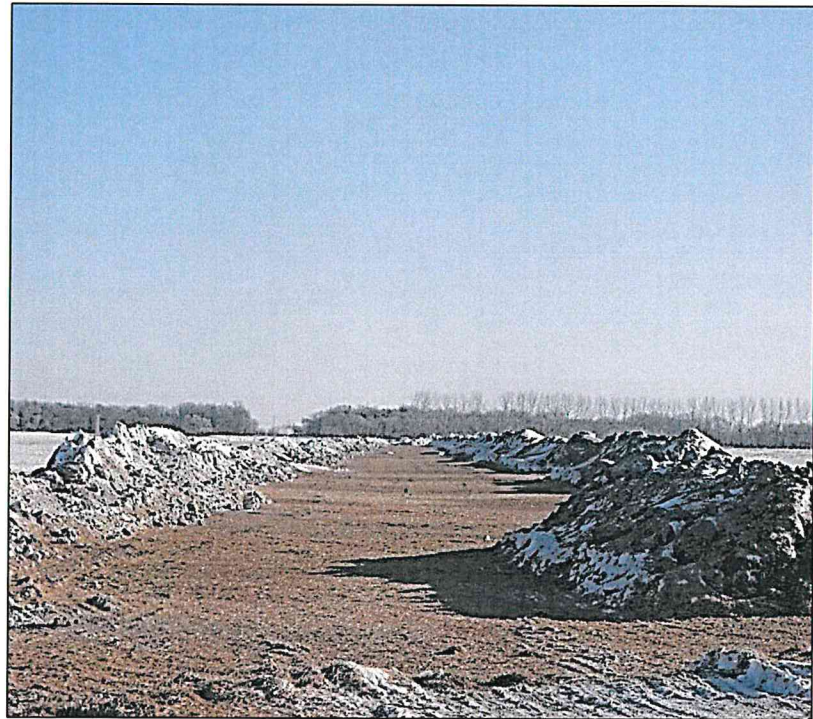
Right-of-Way Prepared for Final Stabilization
