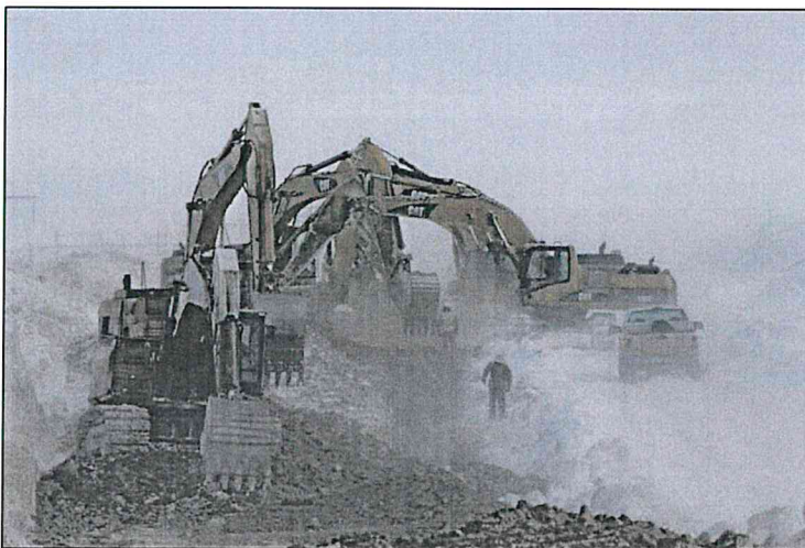
Pipeline Construction in Frozen Conditions
