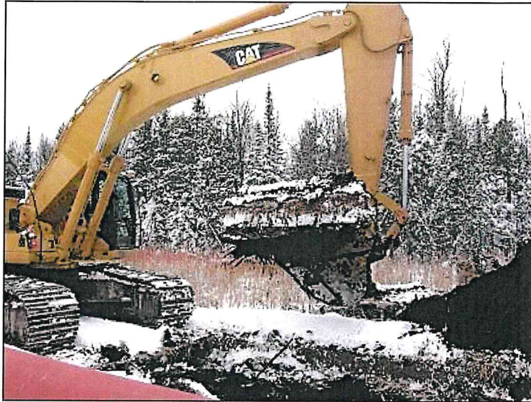
Segregating Frozen Topsoil Layer in Wetland
