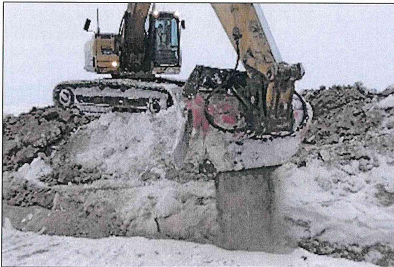
Shaker Equipment Backfilling Trench
