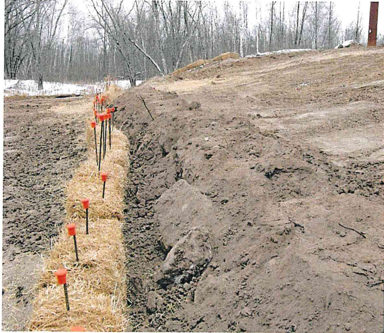
Erosion Control Devices With Protective Caps on Metal Stakes
