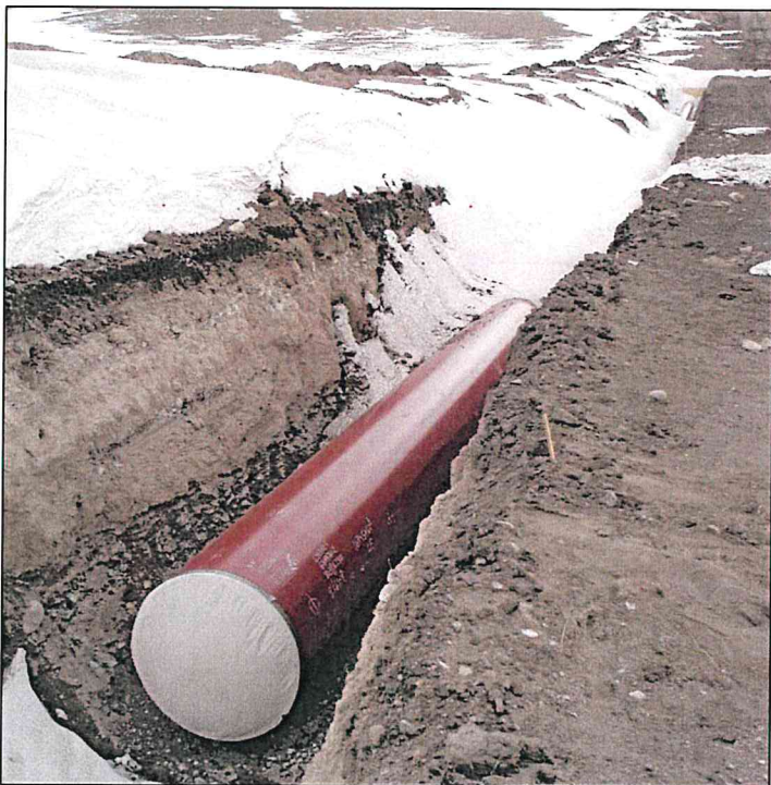
Pipeline Construction in Frozen Conditions
