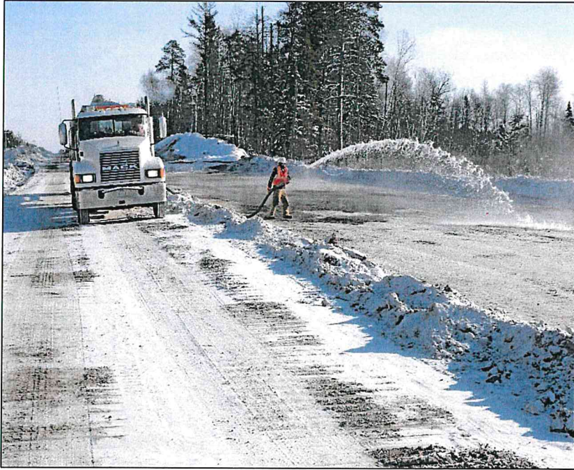
Building the Ice Road
