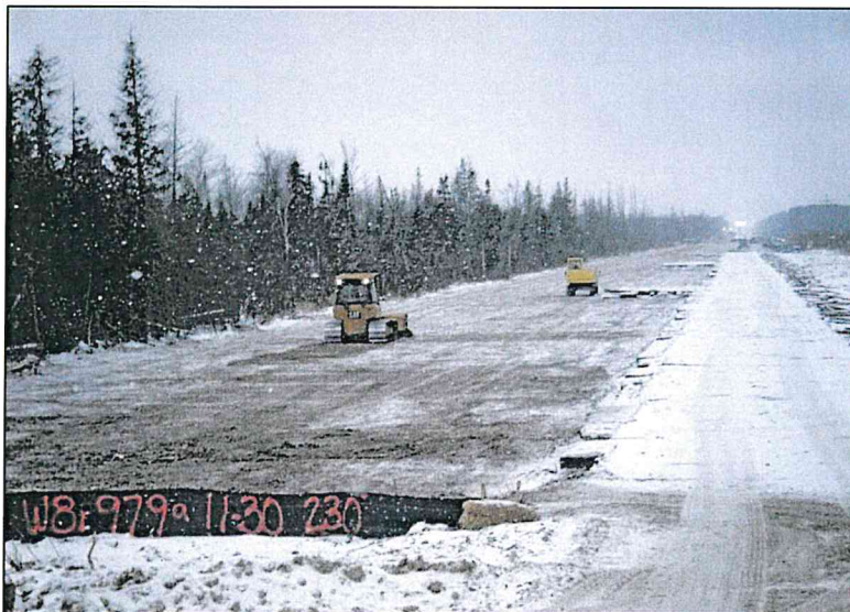
Preparing the Right-of-Way
