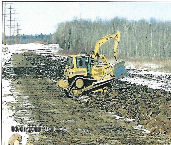
Reducing Frozen Crown Over Backfilled Trench
