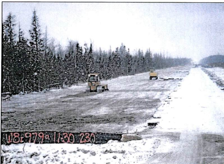
Preparing the Right-of-Way
