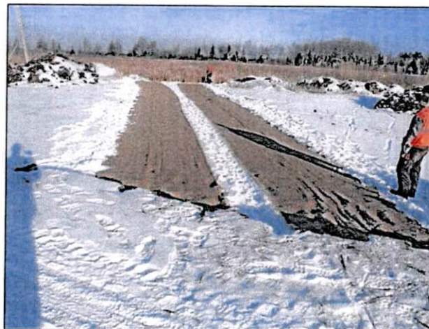
Stabilization of the Right-of-Way
