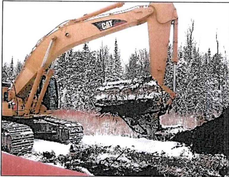
Segregating Frozen Topsoil Layer in Wetland
