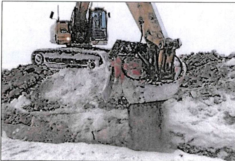
Shaker Equipment Backfilling Trench
