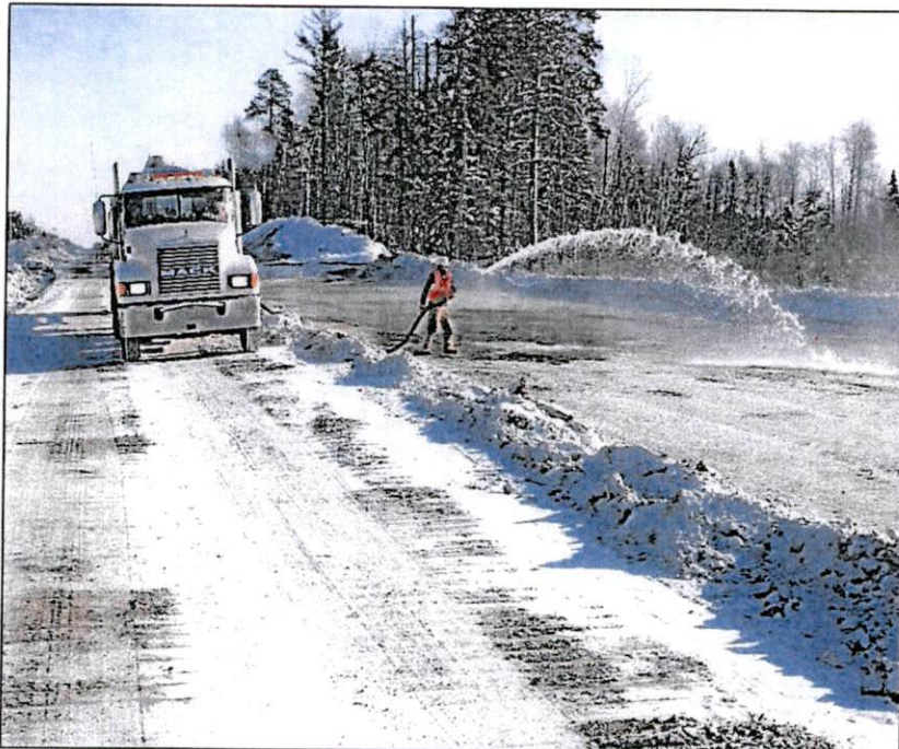
Building the Ice Road
