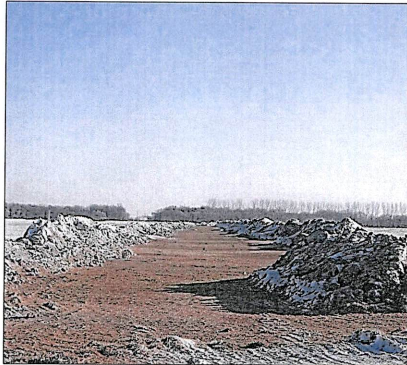
Right-of-Way Prepared for Final Stabilization
