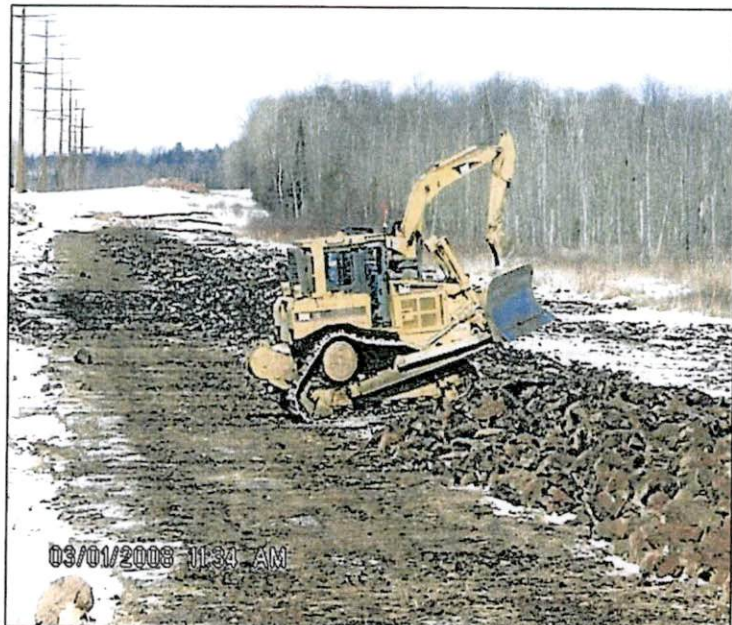
Reducing Frozen Crown Over Backfilled Trench
