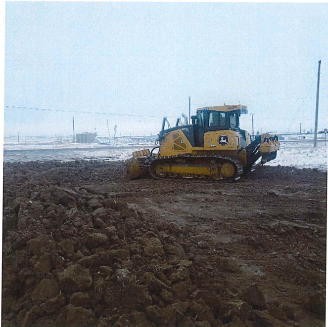
P2 - STA 3+80 BK, Topsoil Removal
