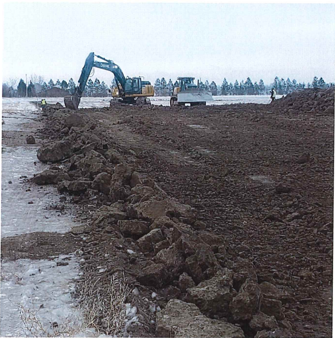
P32 – STA 5+20 Topsoil Removal
