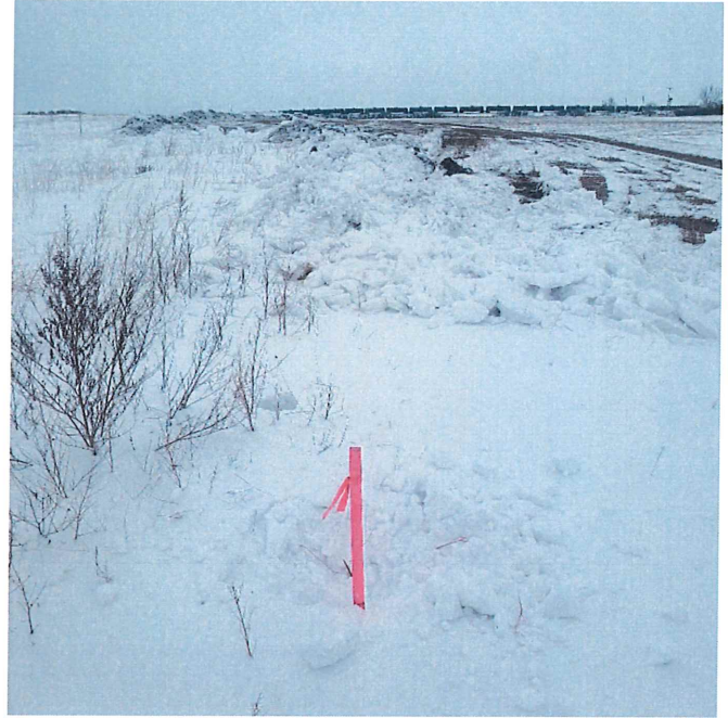
P26 – STA 21+95 BK, End of Snow Removal
