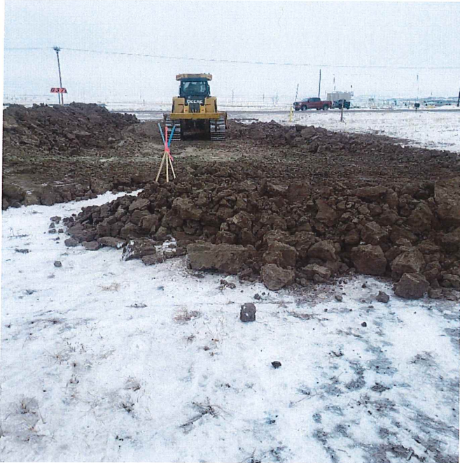
P3 - STA 4+11 BK, Topsoil Removal
