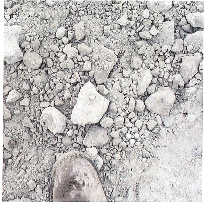
P34 – STA 4+11, Existing Subsoil
