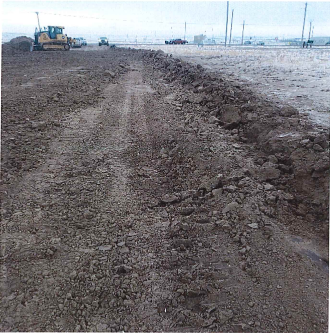
P31 – STA 6+60 Topsoil Removal
