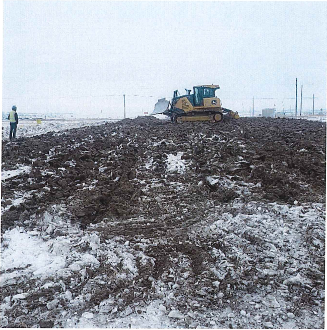
P30 – STA 6+00 BK, Perpendicular Topsoil Ripping
