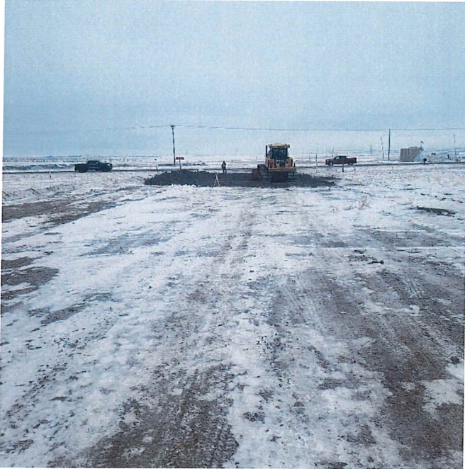
P1 - STA 5+50 BK, Begin Topsoil Removal
