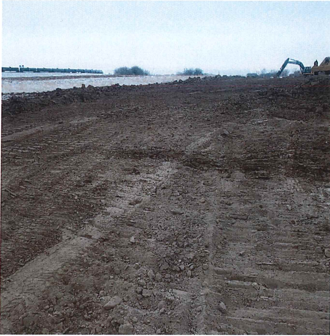
P33 – STA 4+11 AH, Topsoil Removal
