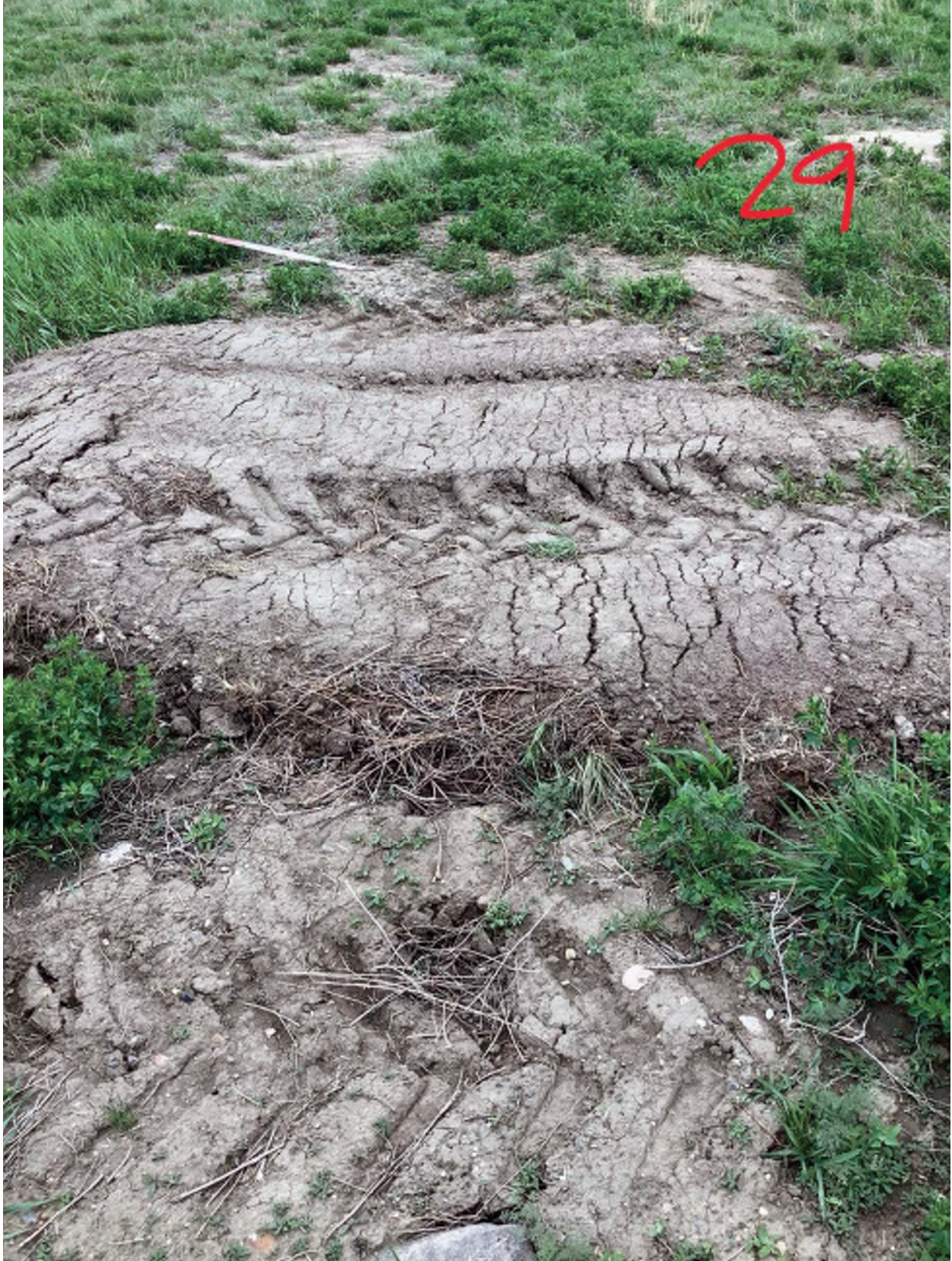
P29 looking W, area where landowner deposited soil to cover trench sink.
