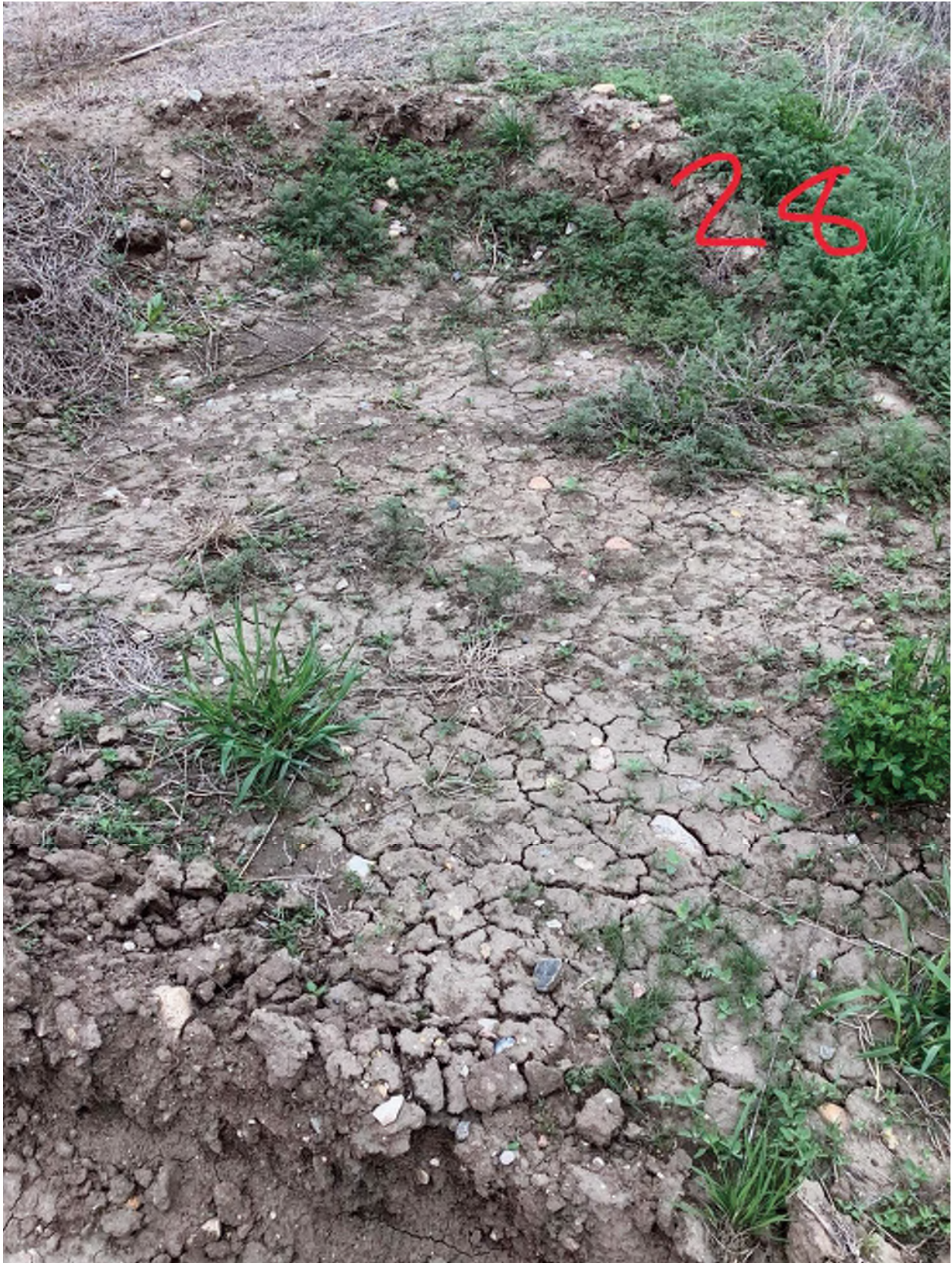
P28 looking S, spot where landowner came in and removed soil to fill trench sink spots.
