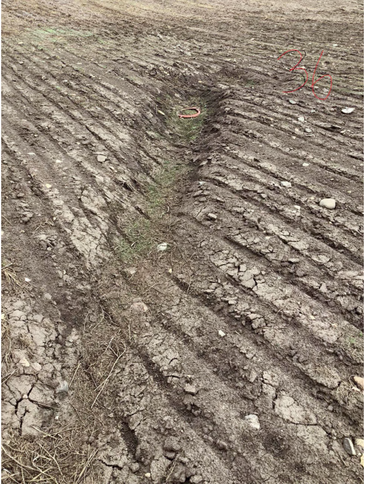
P36 looking NE. Minor trench sink, however landowner was working land anyway.
