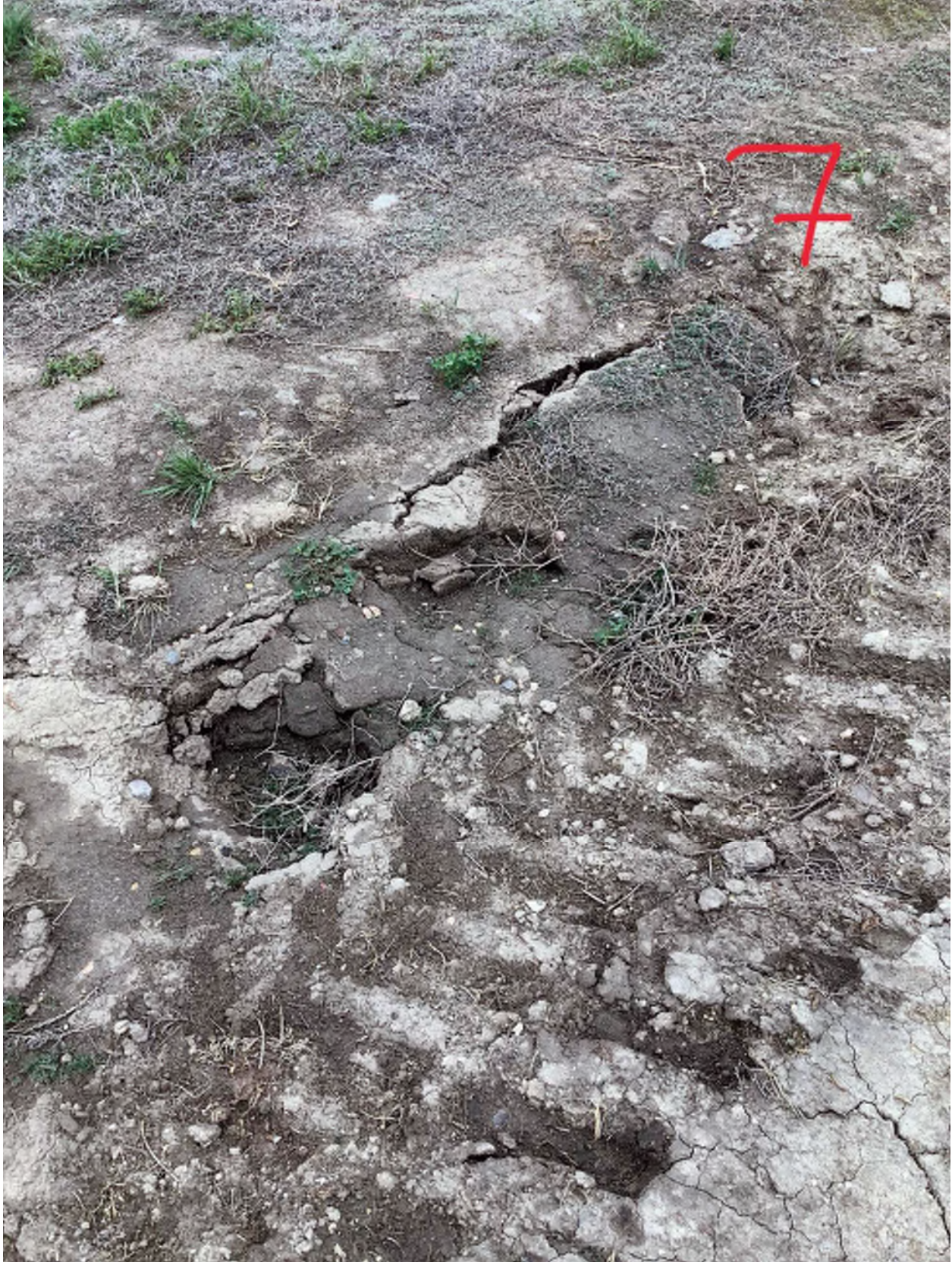
P7: Looking SW, farmer filled in section of trench sinkage, almost no vegetative cover.
