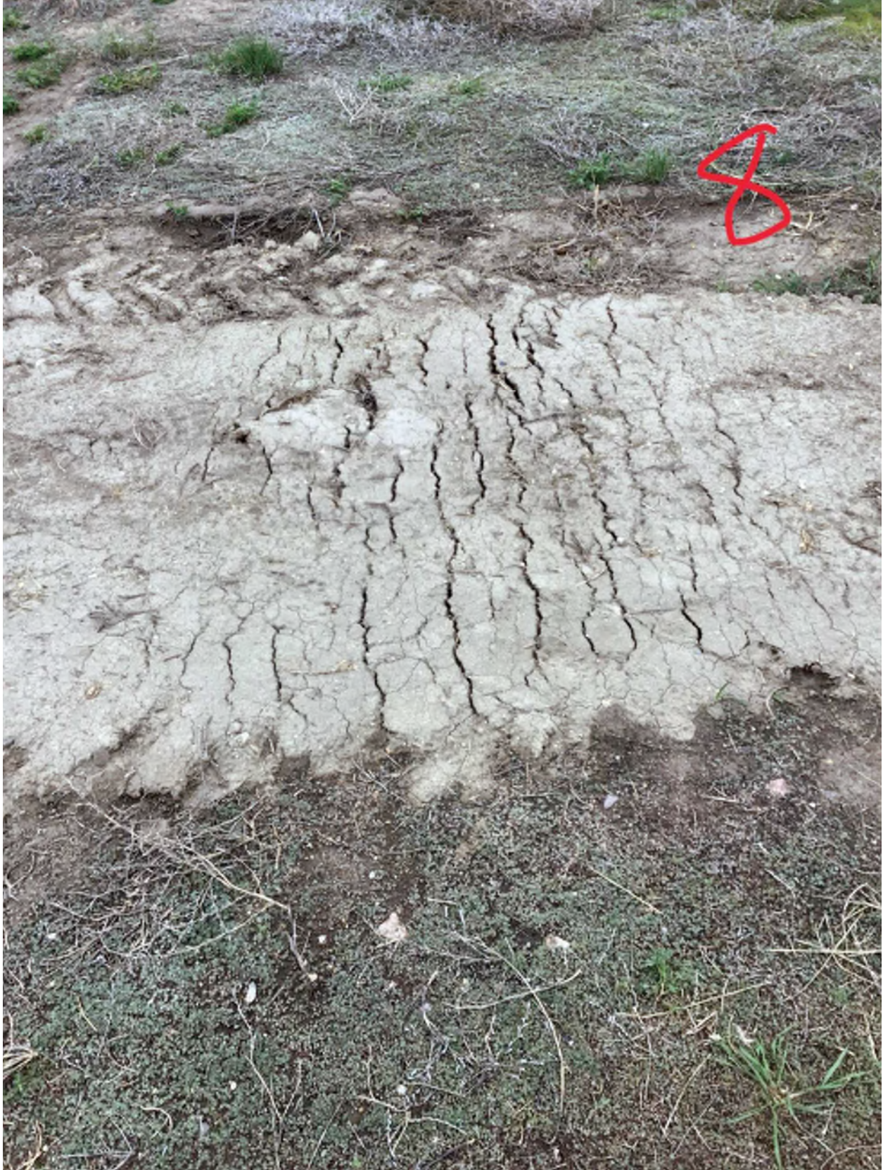
P8 looking S, sinkage remedied by the landowner, notice plant cover adjacent to fill location.
