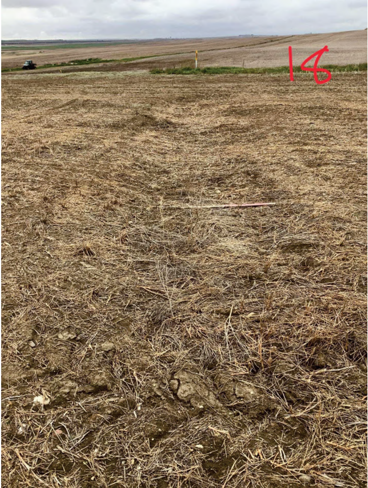
P18 looking NE, minor trench sinkage and substantive crop cover. Landowner has been working the field.
