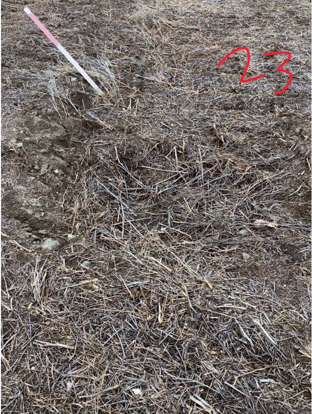
P23 looking NE, localized trench sinkage.
