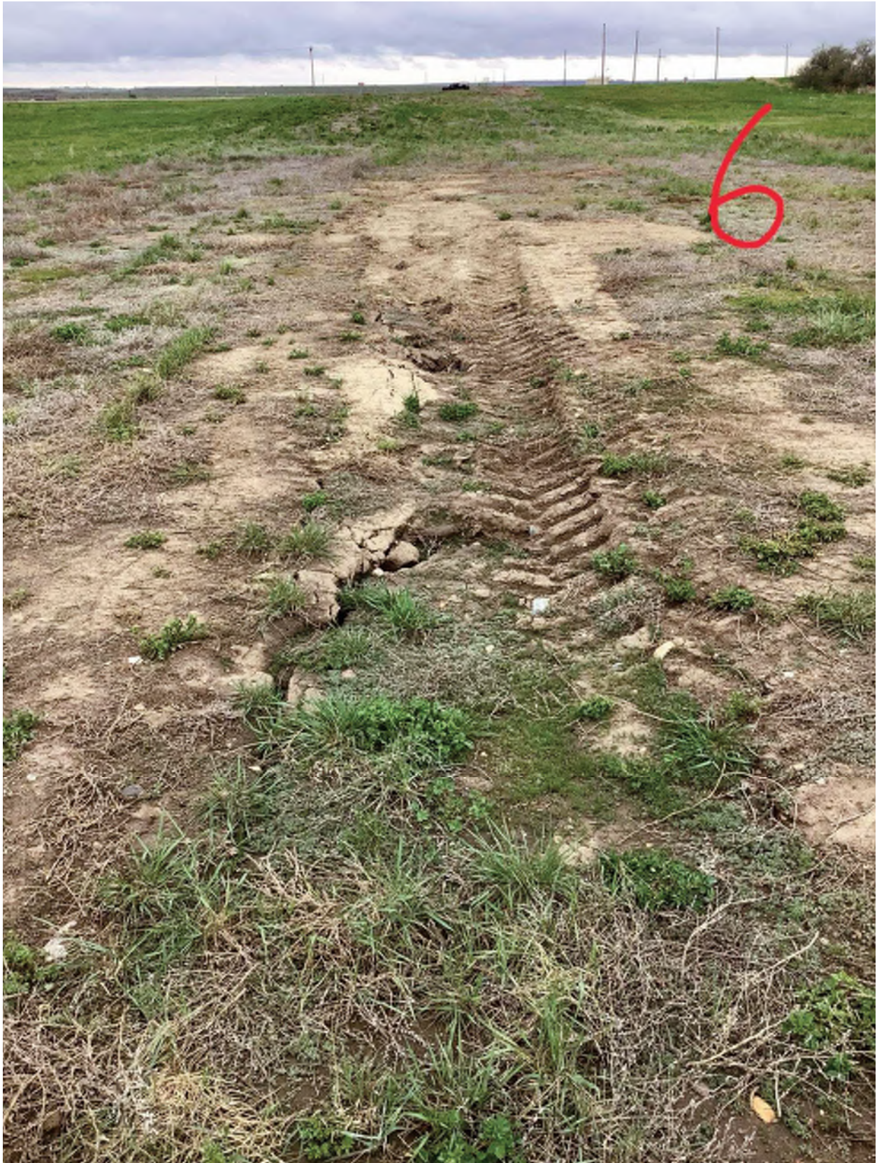
P6: looking West: Area where landowner has filled previous trench sinkage on their own.
