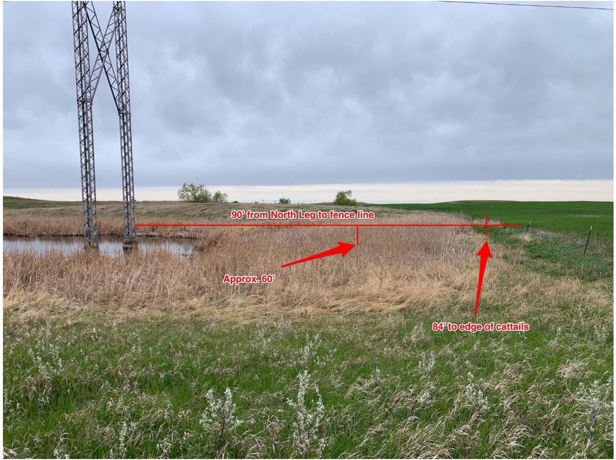
PHOTO OF EXISTING STRUCTURE 597
