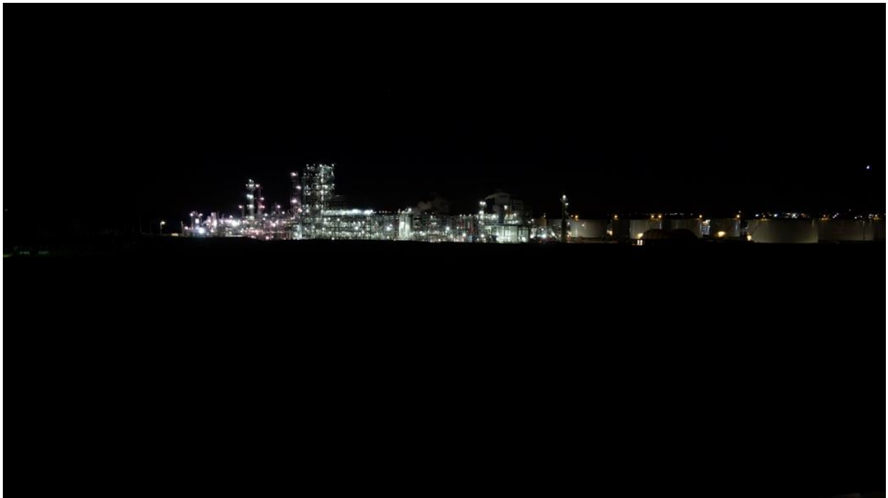
The Renewable Diesel Facility in Dickinson, ND at night
