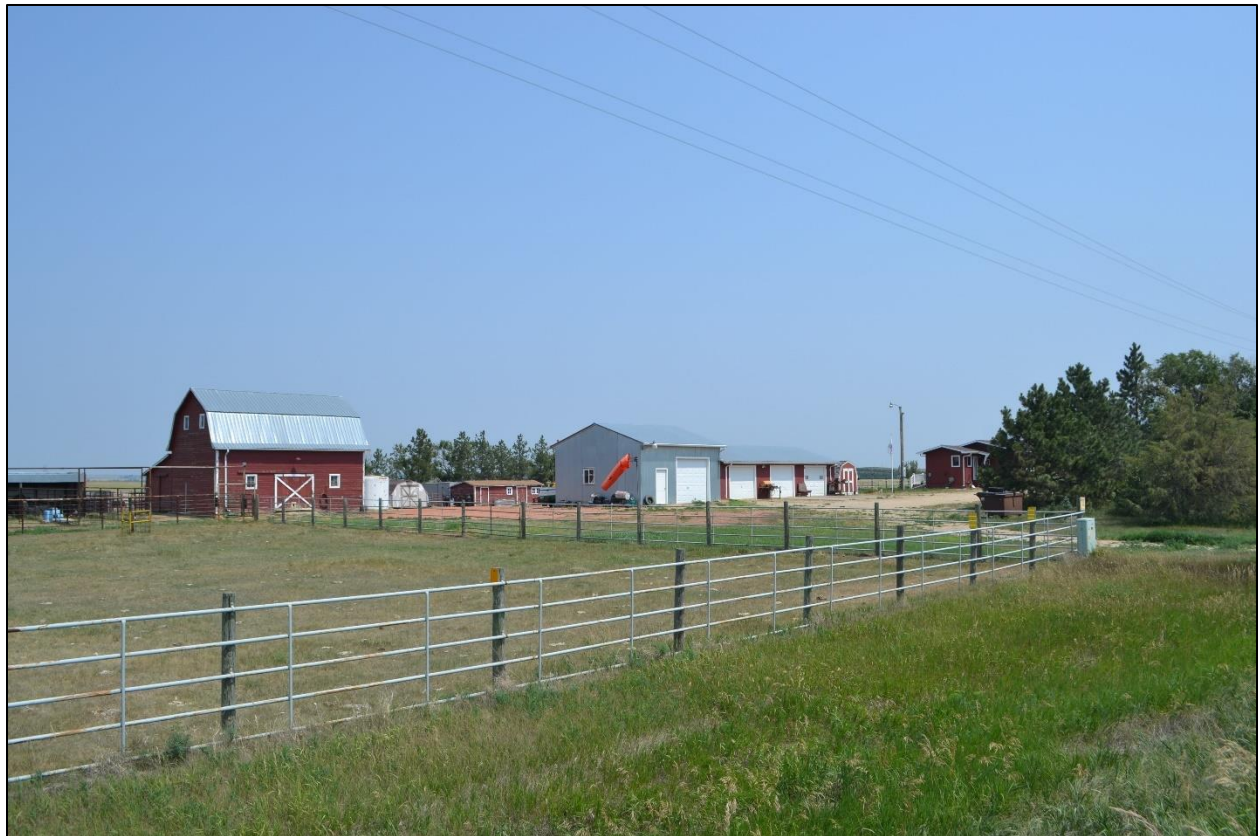
Figure 16. From left, Resources 10f, 10e, 10g, 10h, 10i, 10j, 10d, 10c, and 10b, facing northeast. Photographed by SWCA (H. Curry), July 22, 2021; image has not been altered.
