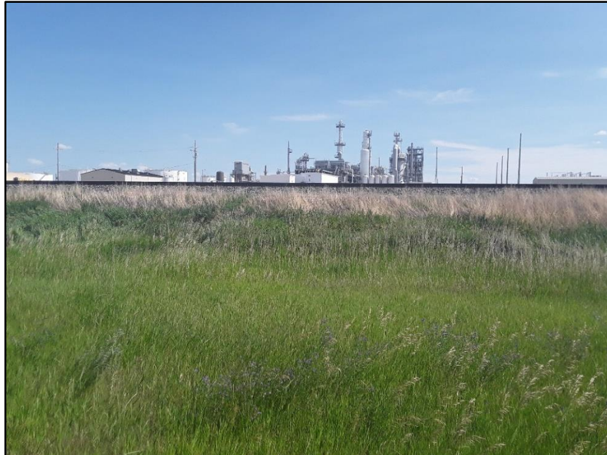
Figure 8. 32SK795 Segment 1 site overview, facing south.
