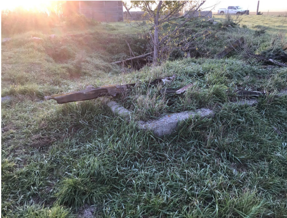
Figure 41. Site 32LO165 Feature 3 overview looking southeast.
