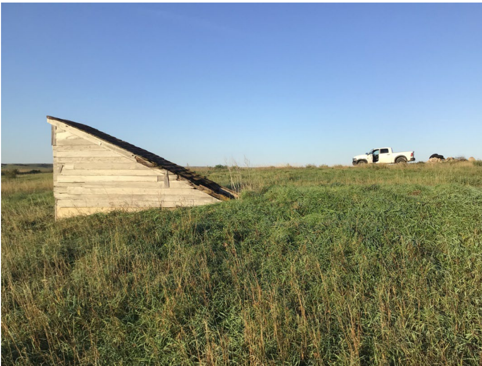
Figure 47. Site 32LO166 Feature 1 tornado shelter looking west.
