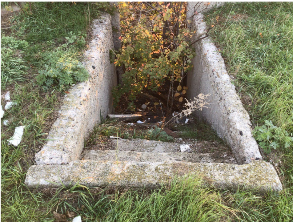
Figure 38. Site 32LO165 Feature 1 close-up of stairs to basement.
