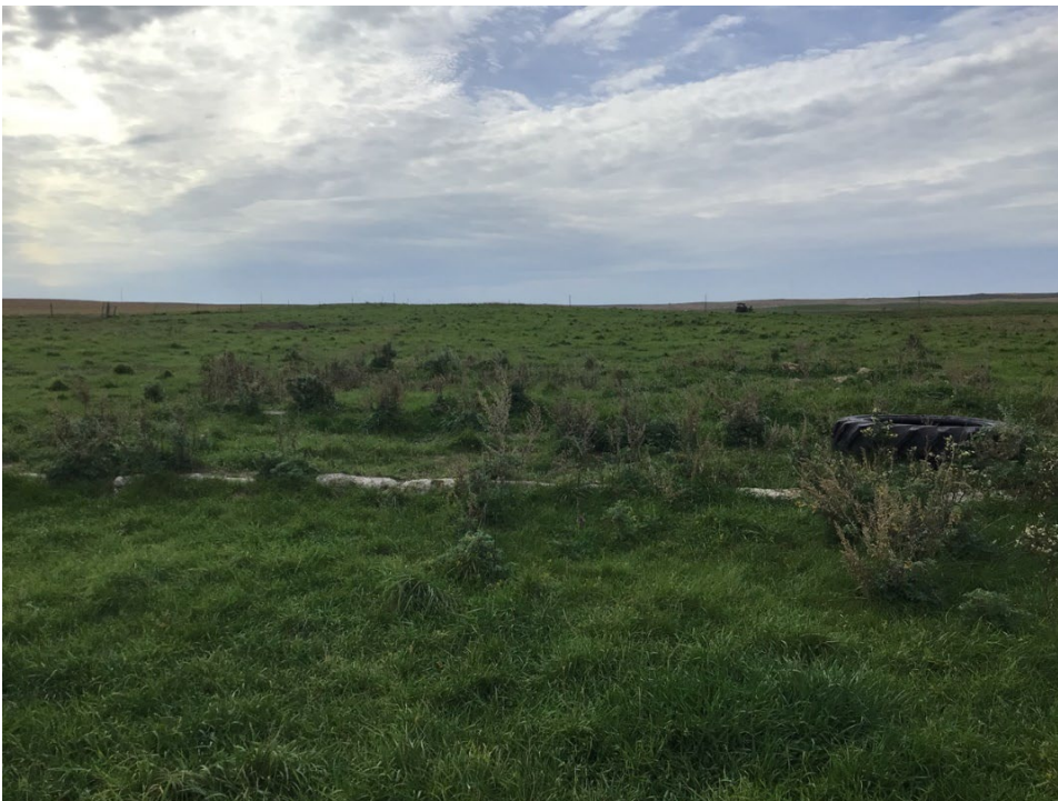
Figure 53. Site 32LO167 Feature 2 overview of outbuilding foundation.
