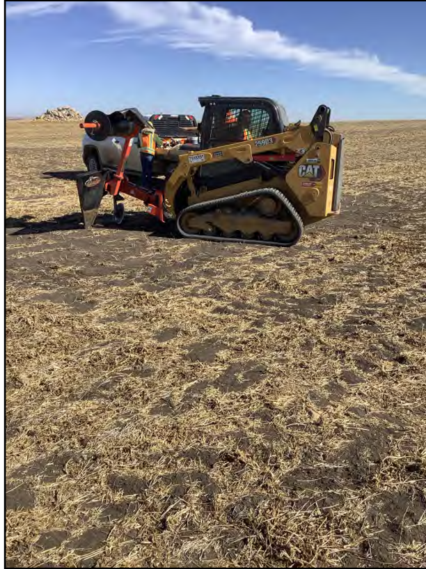
Point 14 Site 3 (structure 65) Crew installing silt fence along NW edge of site.
