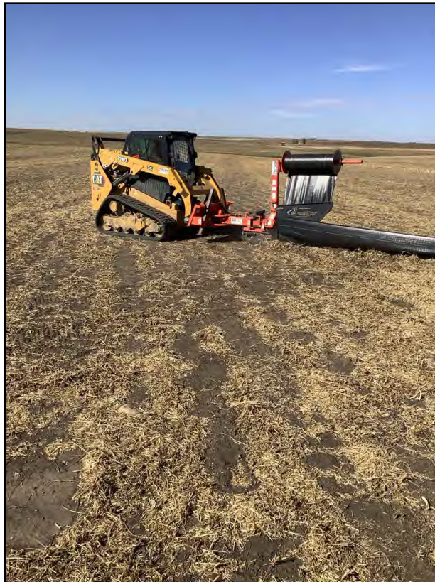
Point 14 Site 3 (structure 65) Crew installing silt fence along NW edge of site.
