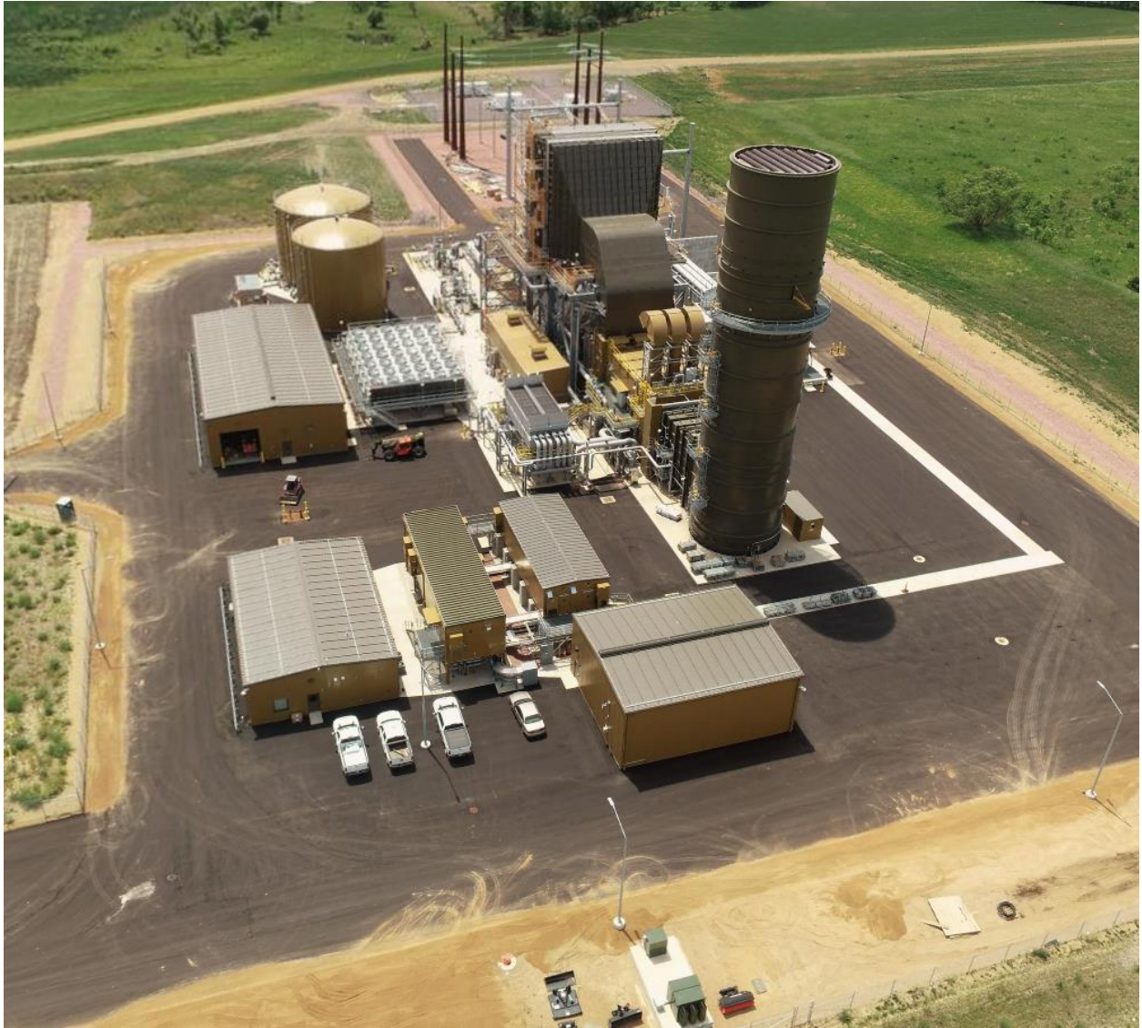
Astoria Station Aerial Photo
