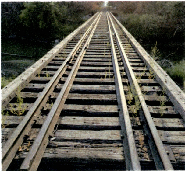
Bridge 11.0 Deck View
