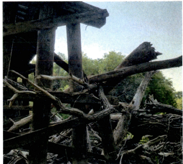
Bridge 11.0 Bent 6 Pile 1
