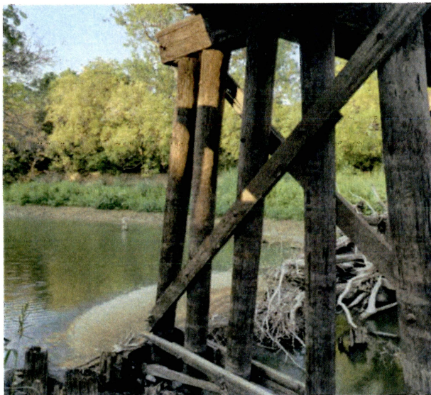
Bridge 11.0 Bent 4 Pile 1
