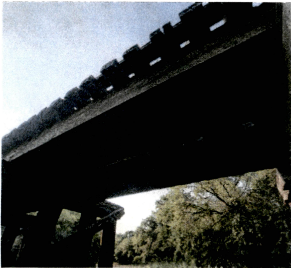
Bridge 11.0 Typical Span
