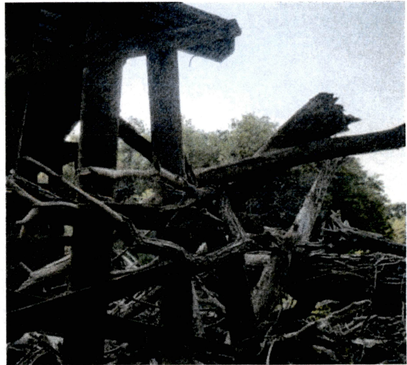
Bridge 11.0 Bent 6 Pile 1
