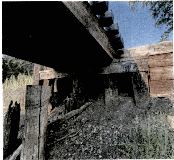
Bridge 11.0 Dump Bent
