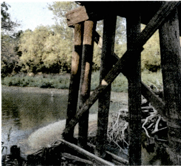
Bridge 11.0 Bent 4 Pile 1
