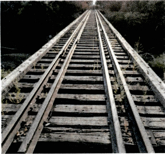
Bridge 11.0 Deck View
