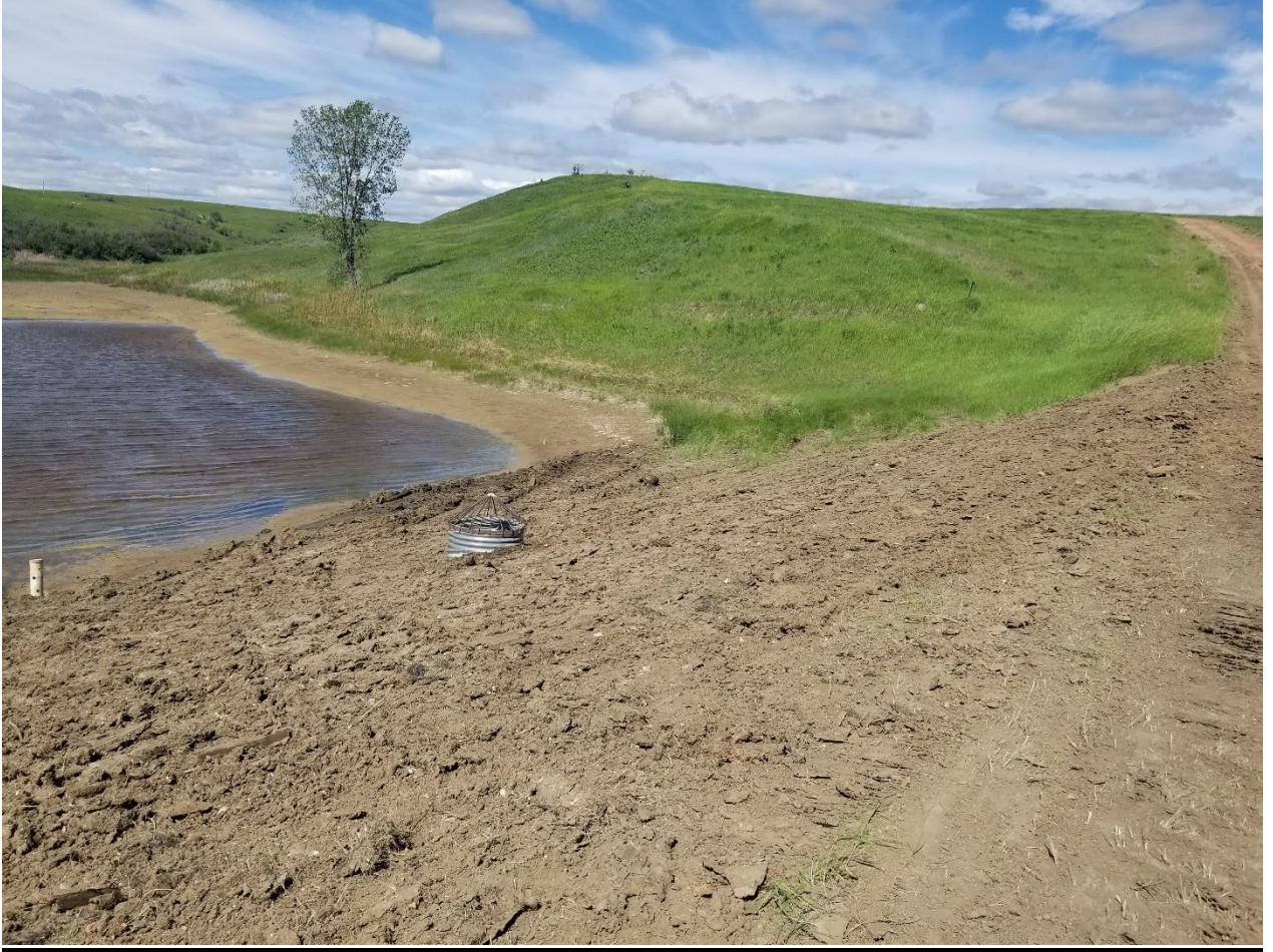
Pond 081 Reconstruction Photo 3
