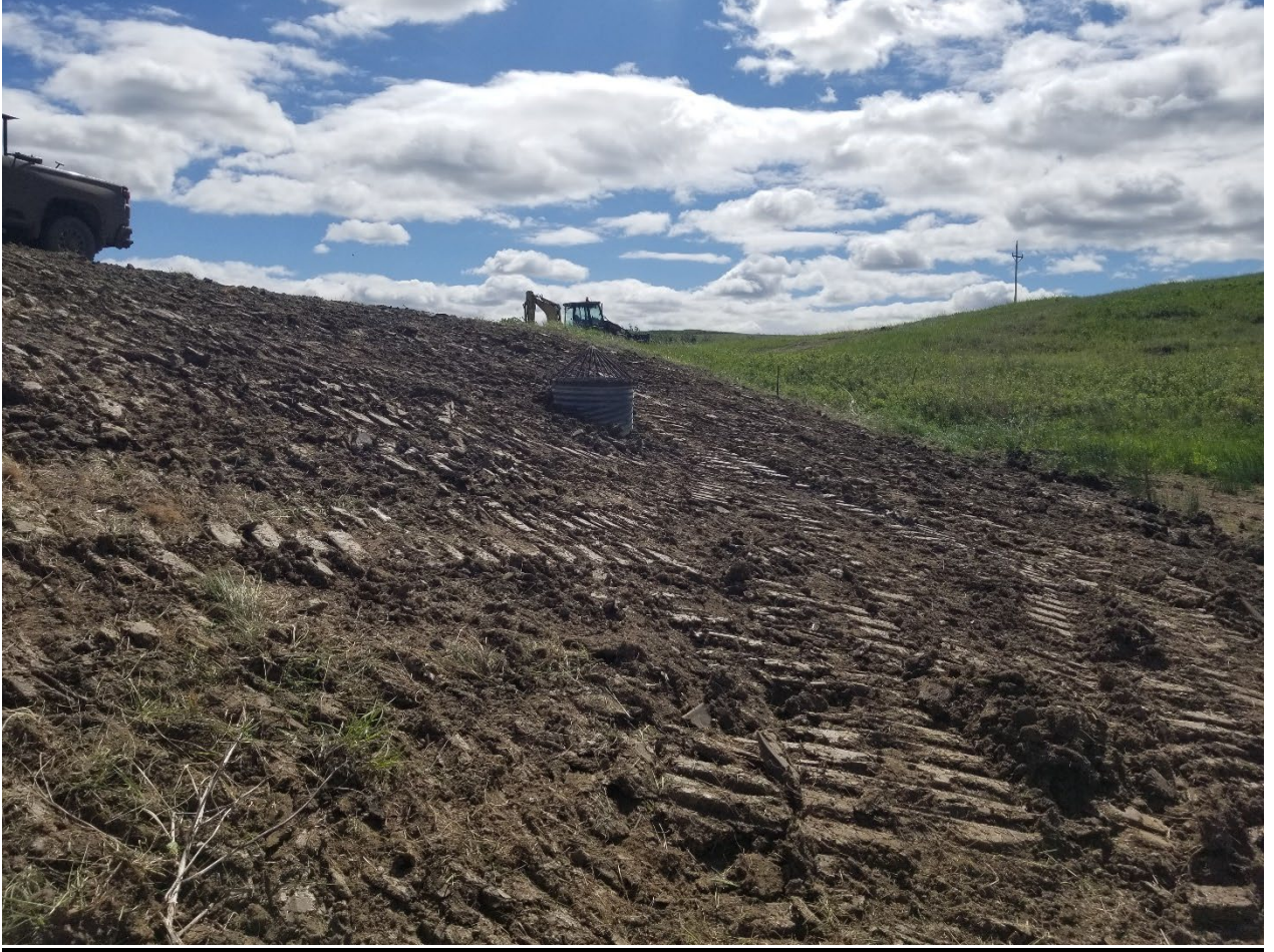
Pond 081 Reconstruction Photo 1
