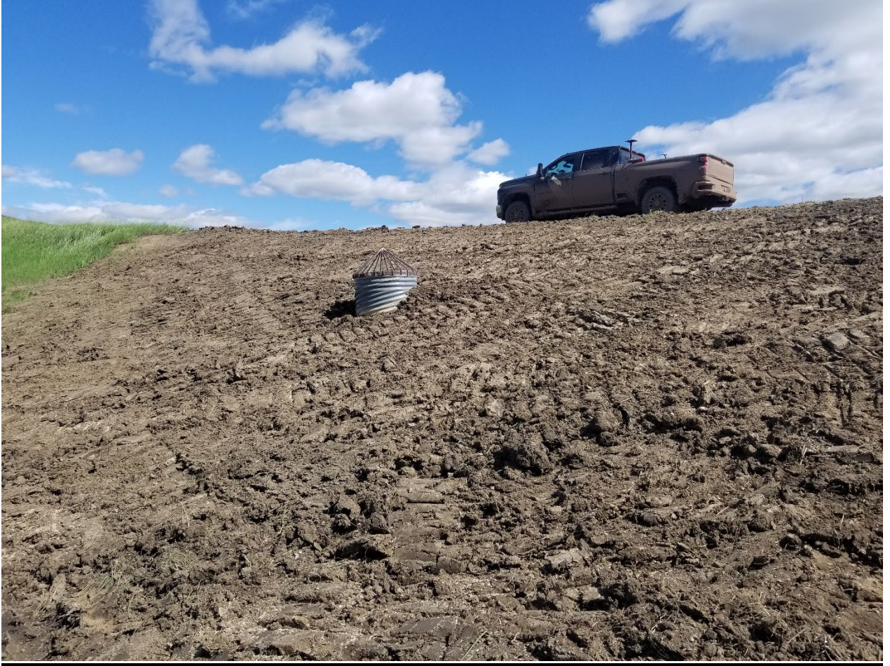
Pond 081 Reconstruction Photo 2
