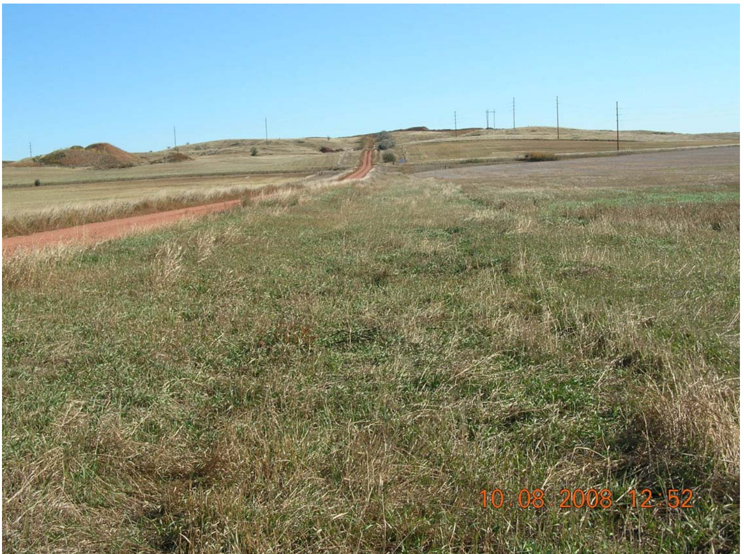
PSC Photo 8 Oct 2008 ... Original road ditch.
