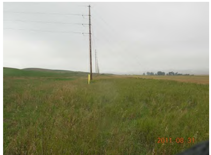
Original diversion ditch with Pond water overflow erosion not visible.
