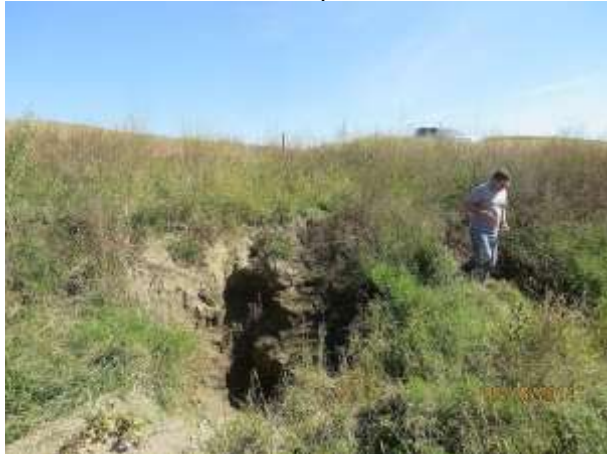
Diversion ditch on 16 Sep 2014
