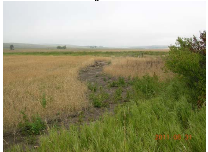
Pond water overflow erosion between original diversion ditch and original road ditch .
