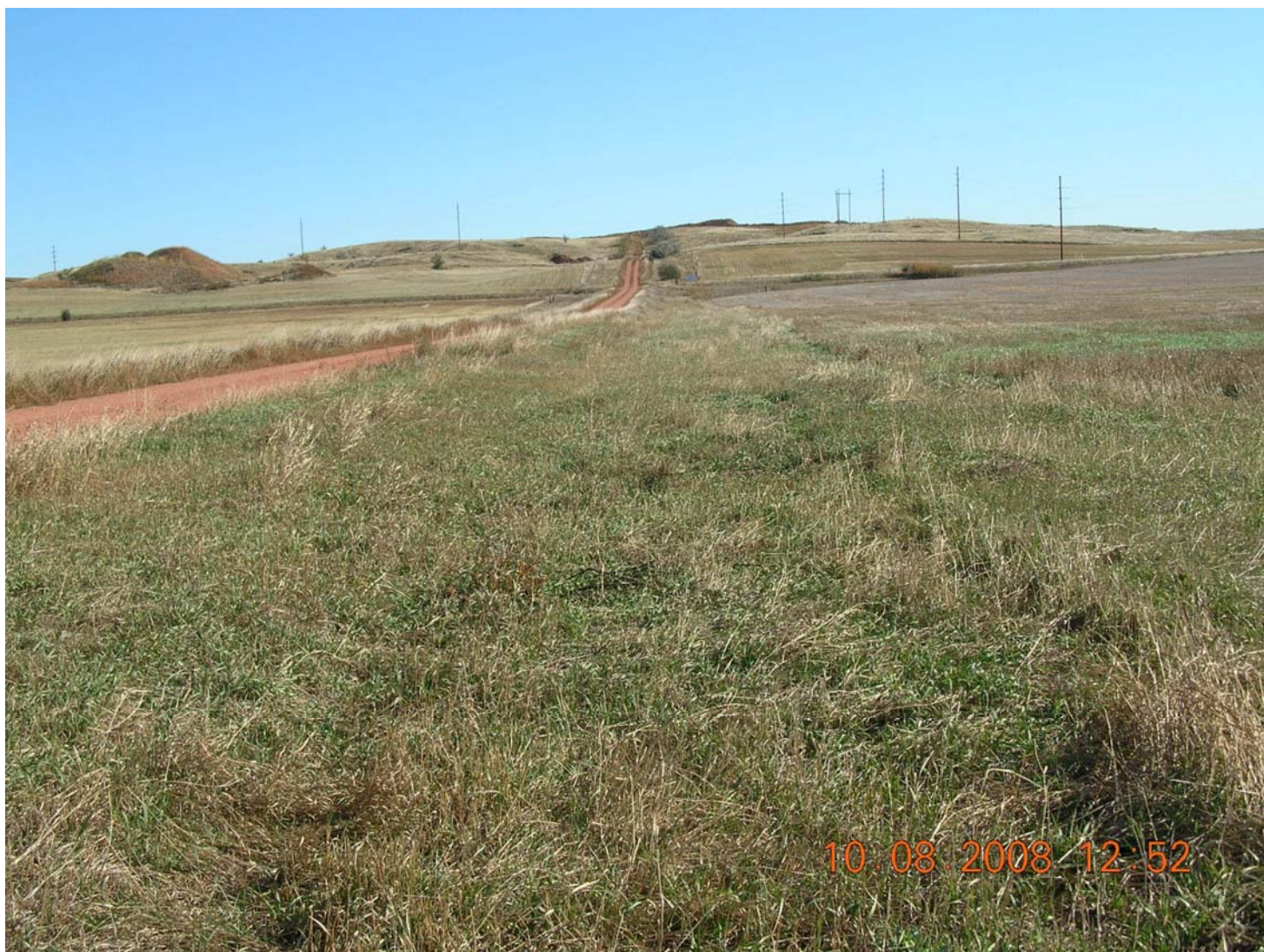
PSC Photo 8 Oct 2008 ... Original road ditch.
