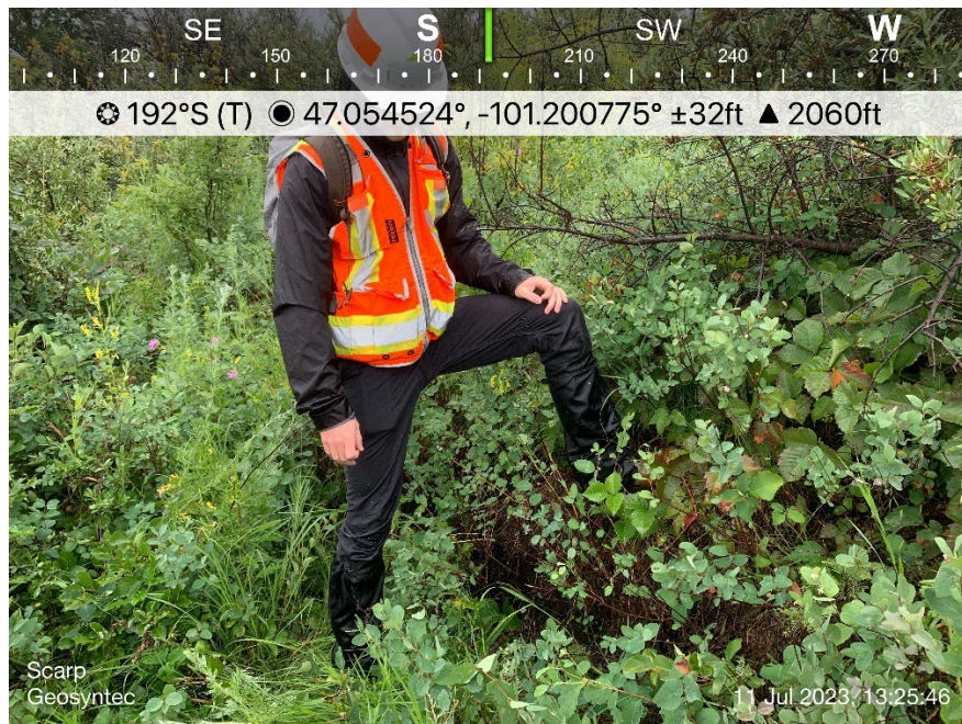
Example of a 2 ft high distinct internal scarp that is associated with the smaller landslide mapped by the NDGS to the southeast of Site #2. The feature is ~50 ft downslope of the proposed pipeline centerline.
