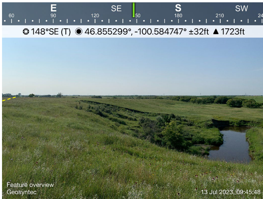
Looking southeast towards Site #15 mapped by the NDGS where recently active landslide morphology was observed approximately 98 ft from the proposed pipeline centerline. The approximate proposed pipeline is located at the far left of the image (dashed yellow line).
