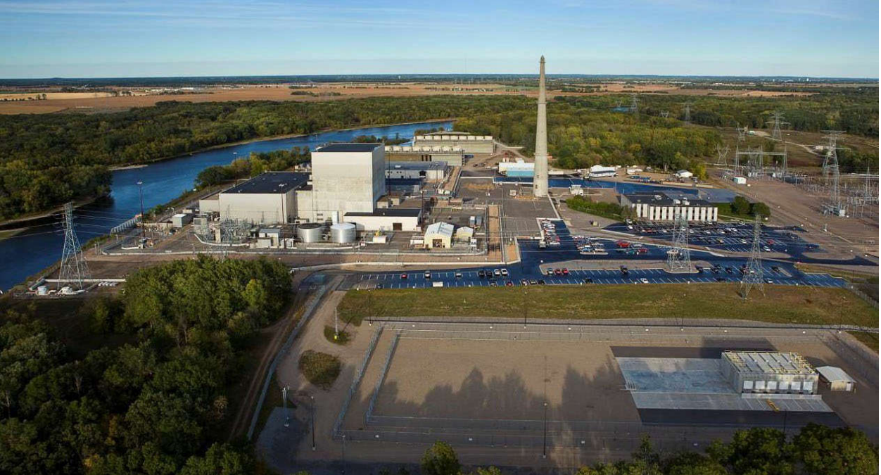
Image 2: Monticello Plant and Existing ISFSI Facilities
