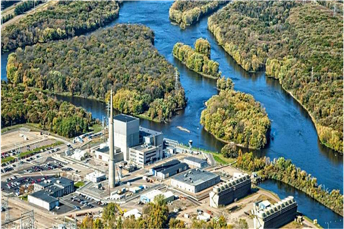
1 Image PP-1: The Monticello Nuclear Generating Plant
