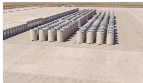
Integrated Storage Partners Andrews, TX
