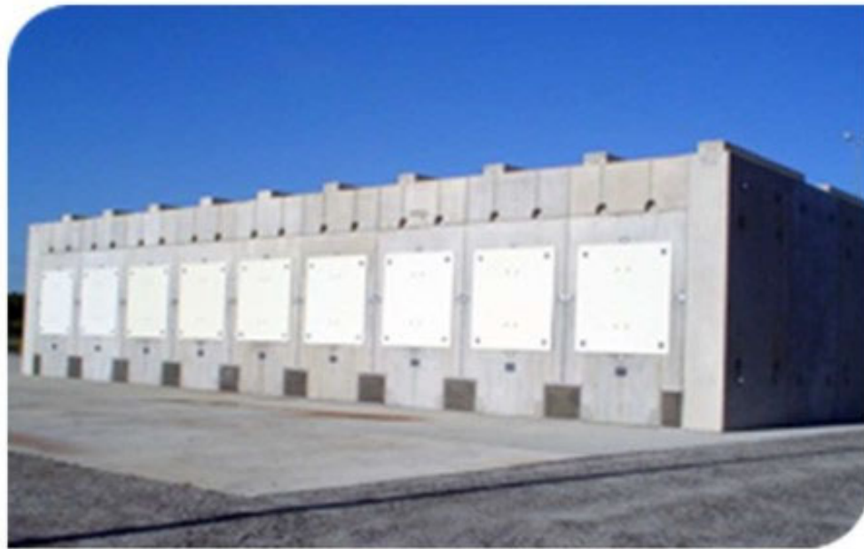
1 Image PP-4: Horizontal Canister System in use at Monticello
