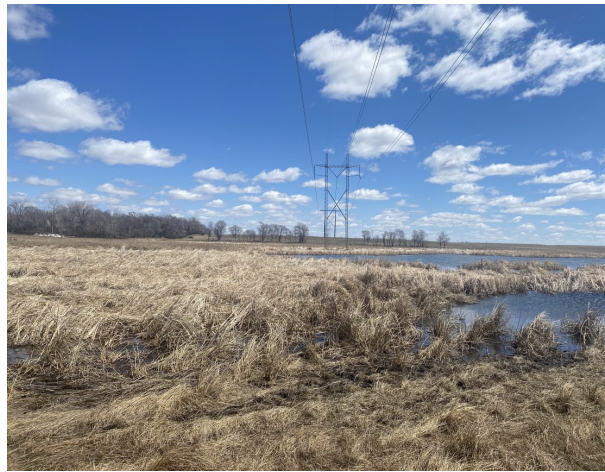
Photo 3: View facing along the utility corridor
