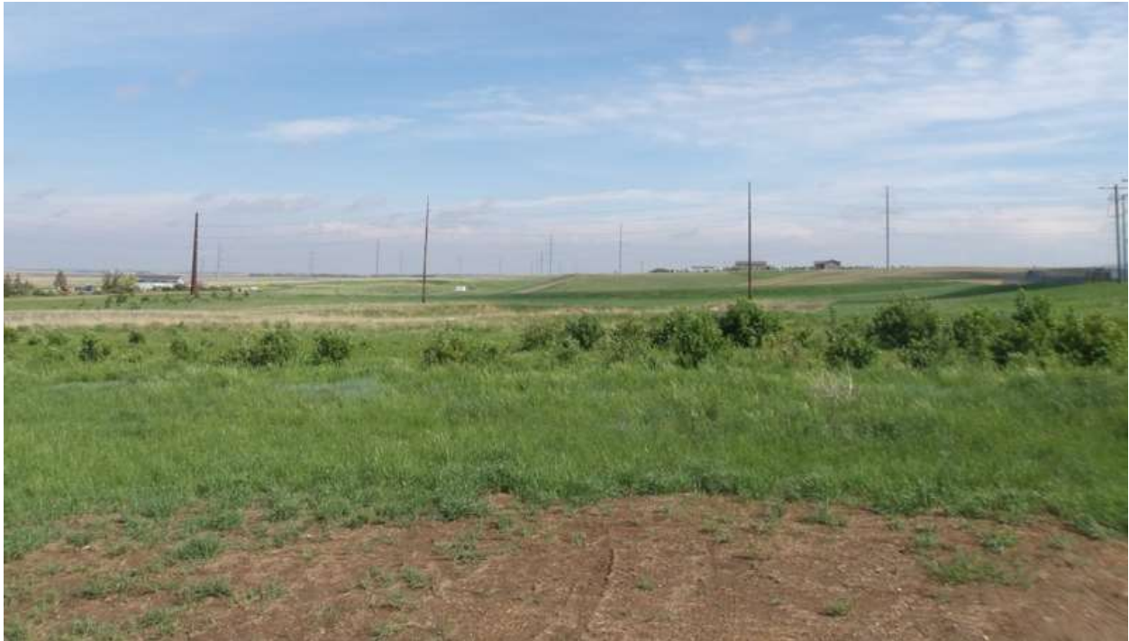
Figure 3: Pioneer to Judson 345 kV transmission line project area, View north (Image #SMT_212, 5/27/23)
