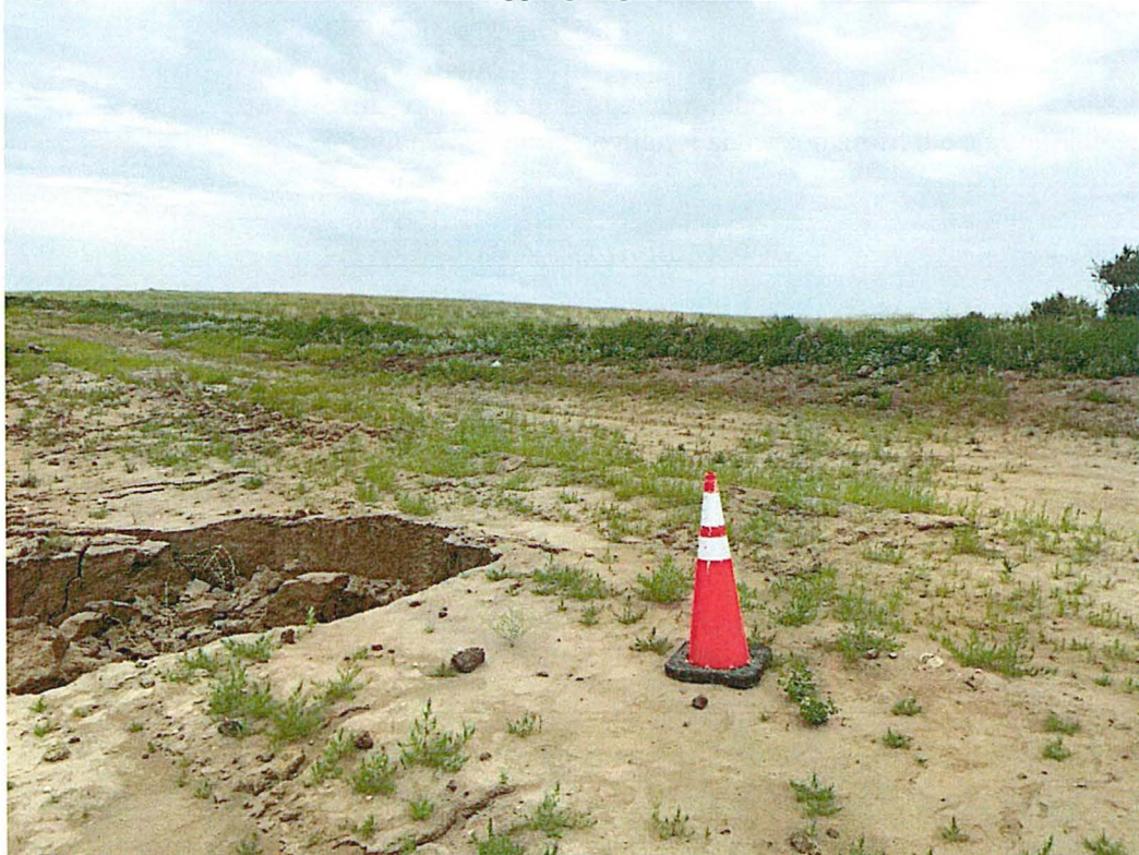
Figure 2. Head cut erosion near the stripping edge in the SW \frac{1}{4} of Section 25.
