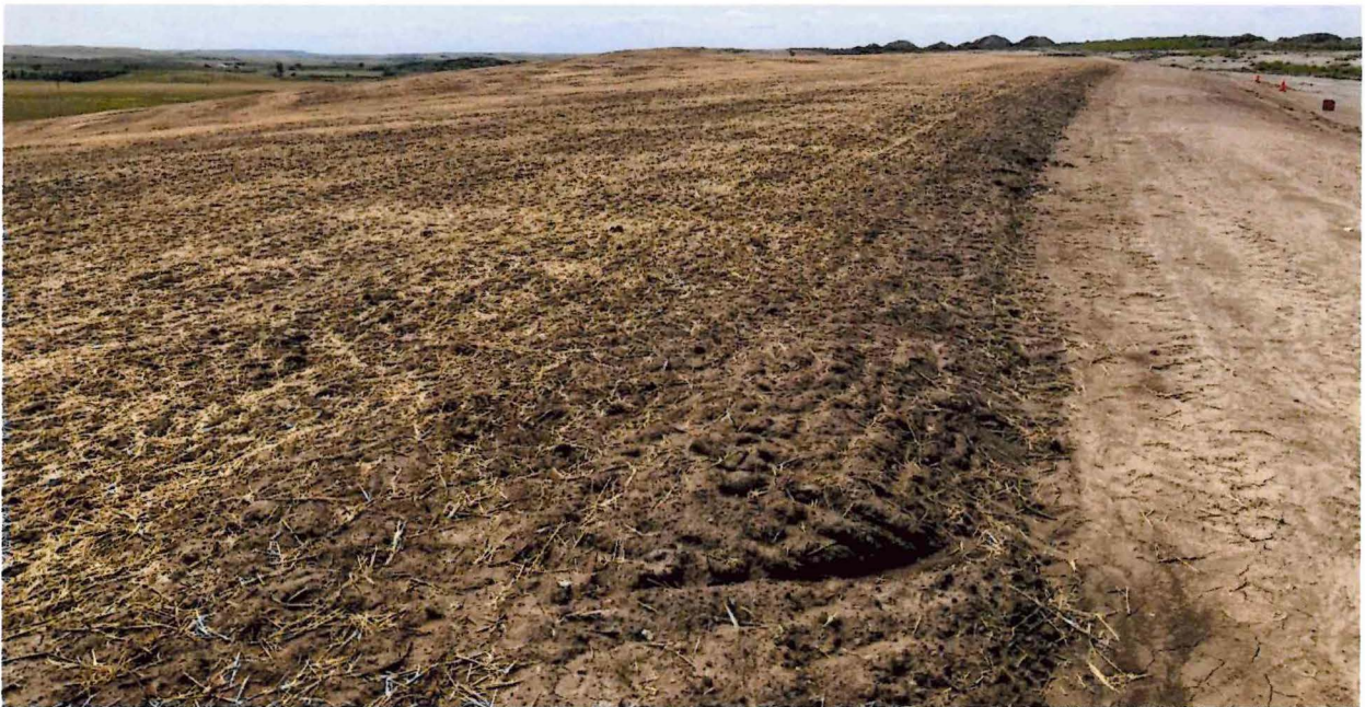
Figure 3: Grade approval COY-035, located in Section 6 and approved 5/9/2023, has been respread with SPGM, seeded with oats, and mulched.
