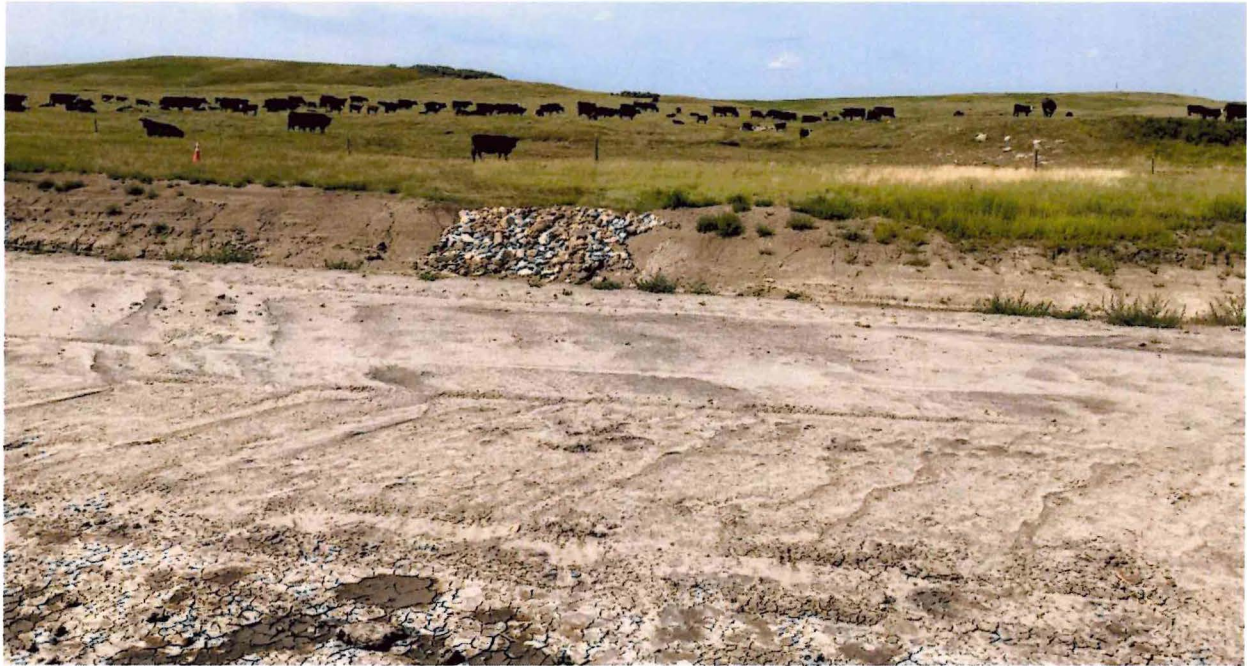
Figure 3: Grade approval COY-035, located in Section 6 and approved 5/9/2023, has been respread with SPGM, seeded with oats, and mulched.
