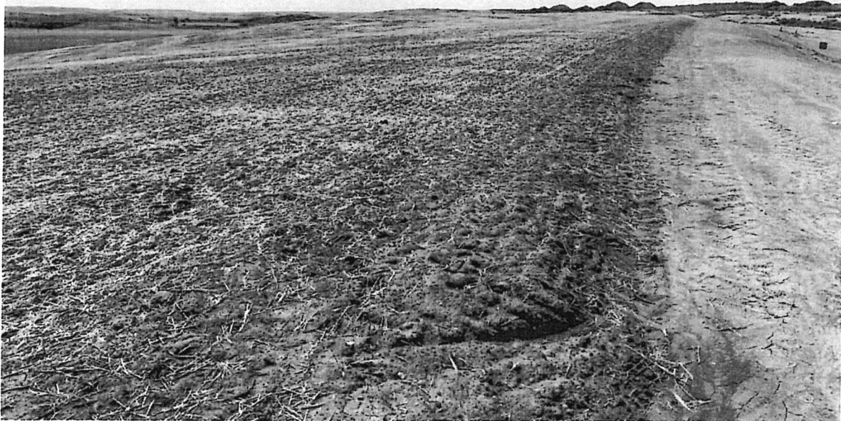
Figure 3: Grade approval COY-035, located in Section 6 and approved 5/9/2023, has been respread with SPGM, seeded with oats, and mulched.
