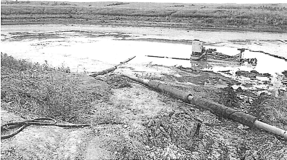
Figure 2. Head cut erosion near the stripping edge in the SW¼ of Section 25.
