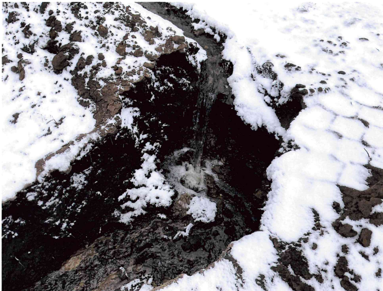
Figure 2 – A head cut and plunge pool that has formed on the east edge of grade approval Gold-01-2022 in Permit KRSB-8603.
