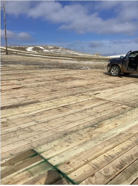
Point 1, Structure #366-057 site layout. Example of matting in use for site disturbance limitation
