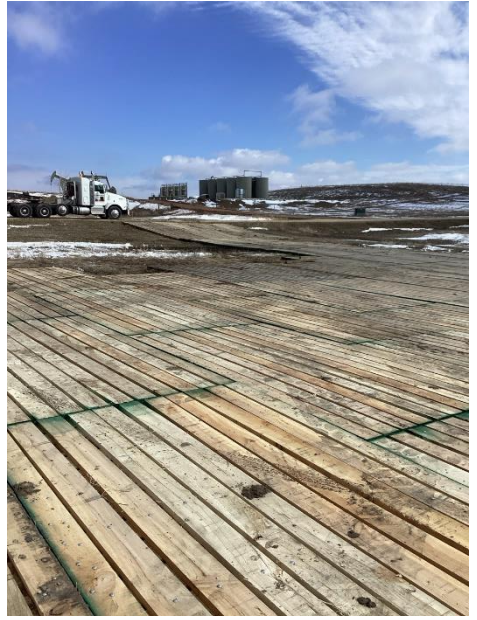
Point 1, Structure #366-057 site layout. Example of matting in use for site disturbance limitation
