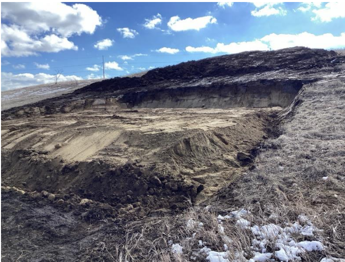
Point 16, Structure #336-058. Finished pad after topsoil and grading complete
