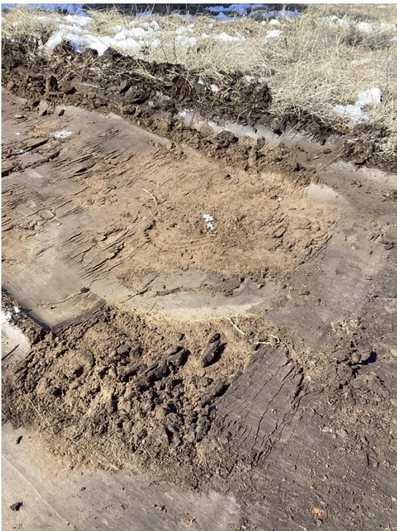
Point 4, Structure # 366-058. Topsoil removal depth shallow at approx. 4"
