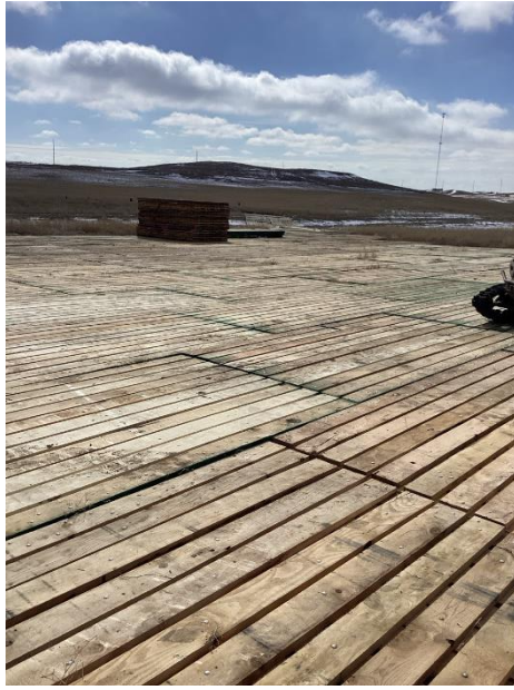
Point 1, Structure #366-057 site layout. Example of matting in use for site disturbance limitation
