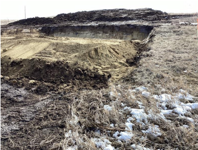
Point 15, Structure #338-058. Drainage ditch cut along pad bottom
