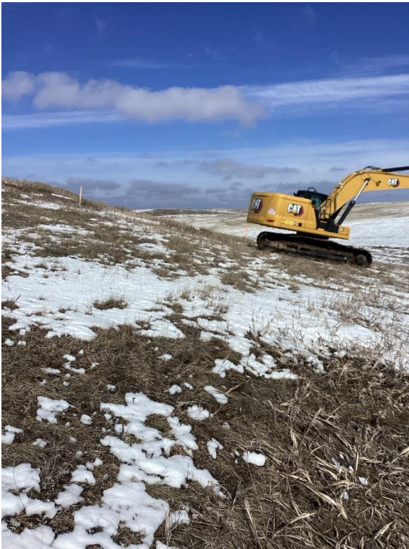
Point 3, Structure #366-058. Start of topsoil removal
