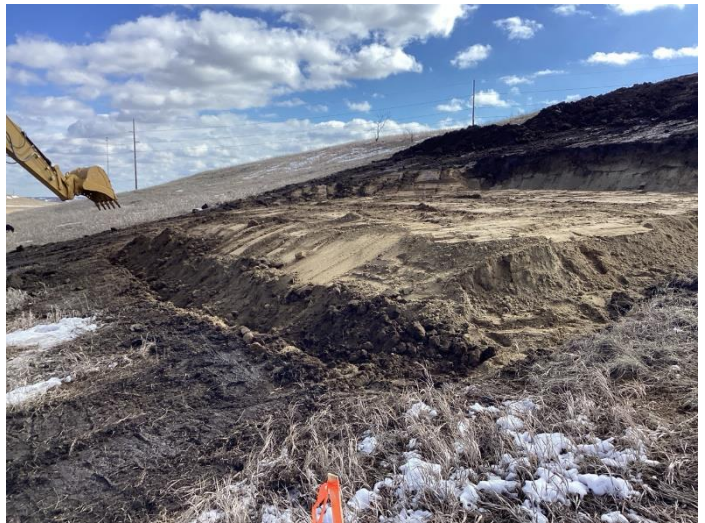
Point 16, Structure #336-058. Finished pad after topsoil and grading complete
