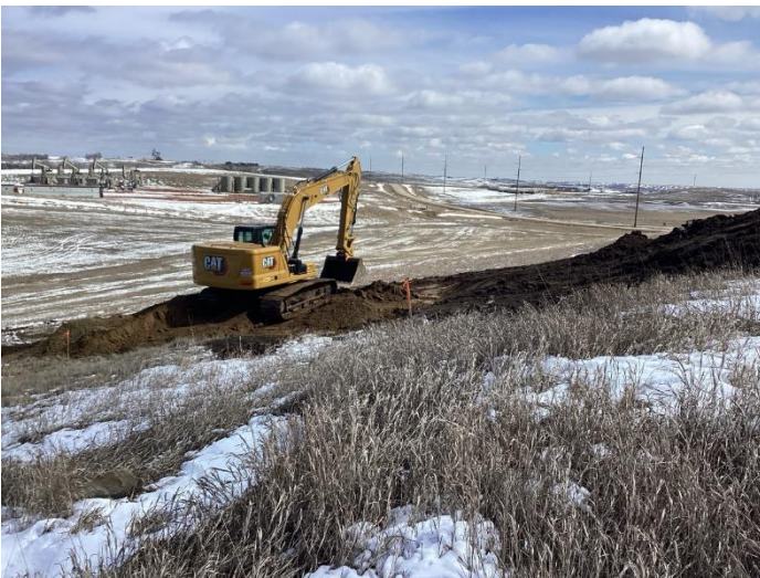
Point 14, Structure #338-058. Pad construction from east side
