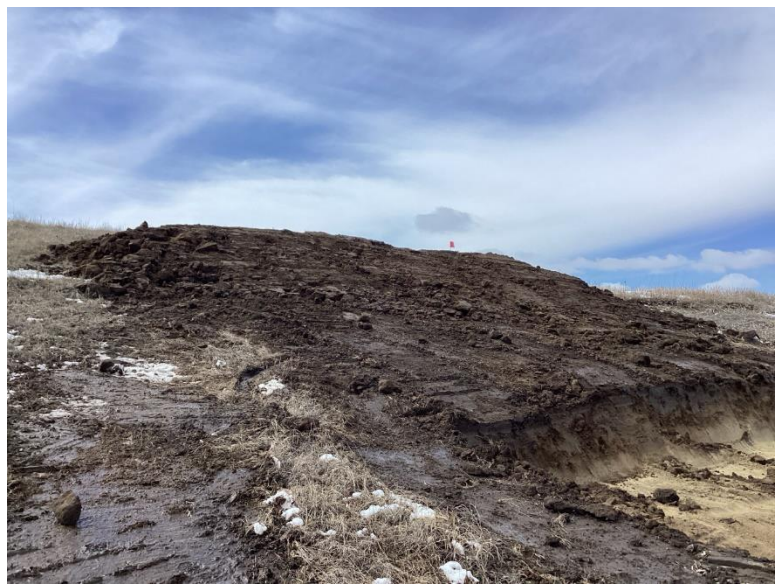
Point 9, Structure #366-058. Finished topsoil storage pile
