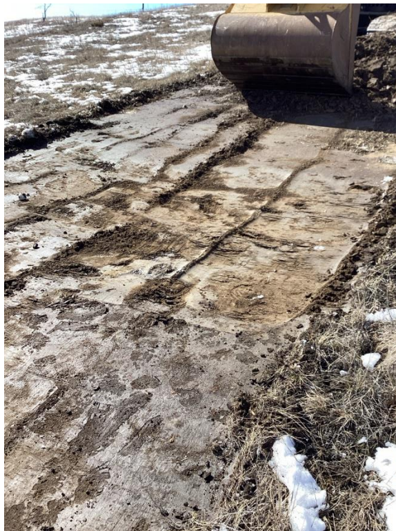
Point 4, Structure # 366-058. Topsoil removal depth shallow at approx. 4"
