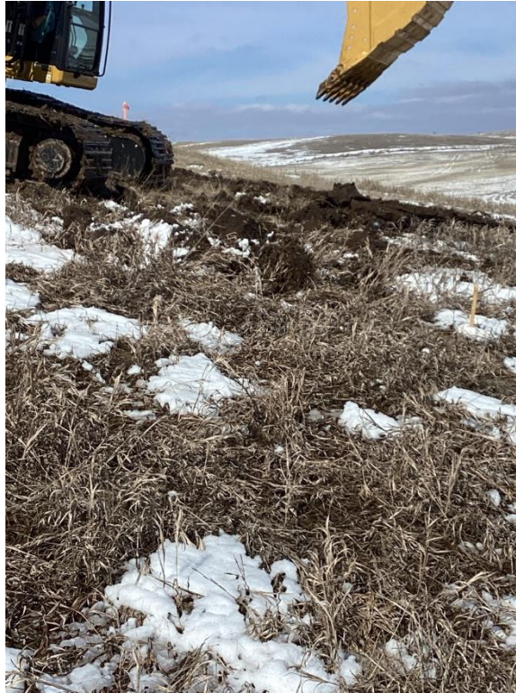
Point 5, Structure #366-058. Broken up topsoil with tooth bucket
