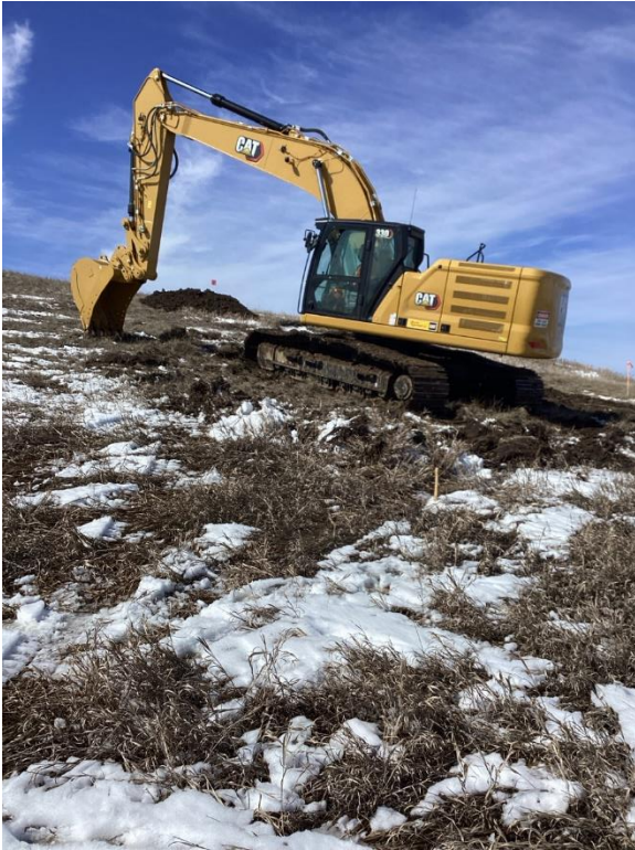
Point 5, Structure #366-058. Broken up topsoil with tooth bucket
