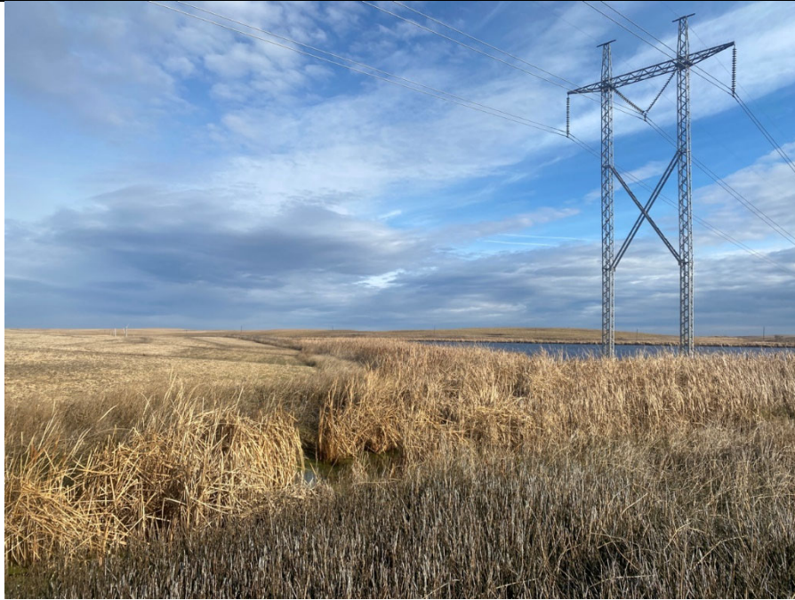
Photo 19: View northeast of the typical landscape present within the Structure #618 corridor. Flat landscape with a mix of wetland and cropland. Wetland/open water located within drainage to the east.
