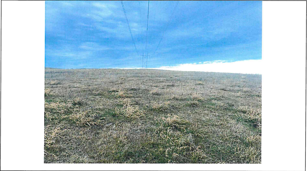
Photo 7: View east of the typical landscape present within the Structure #212 corridor. Gently rolling hills upland grassland landscape, land use is pasture.
