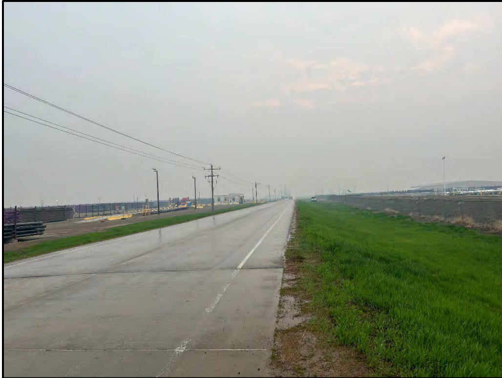
Photograph 1. View looking east down the Survey Corridor from the western start.
