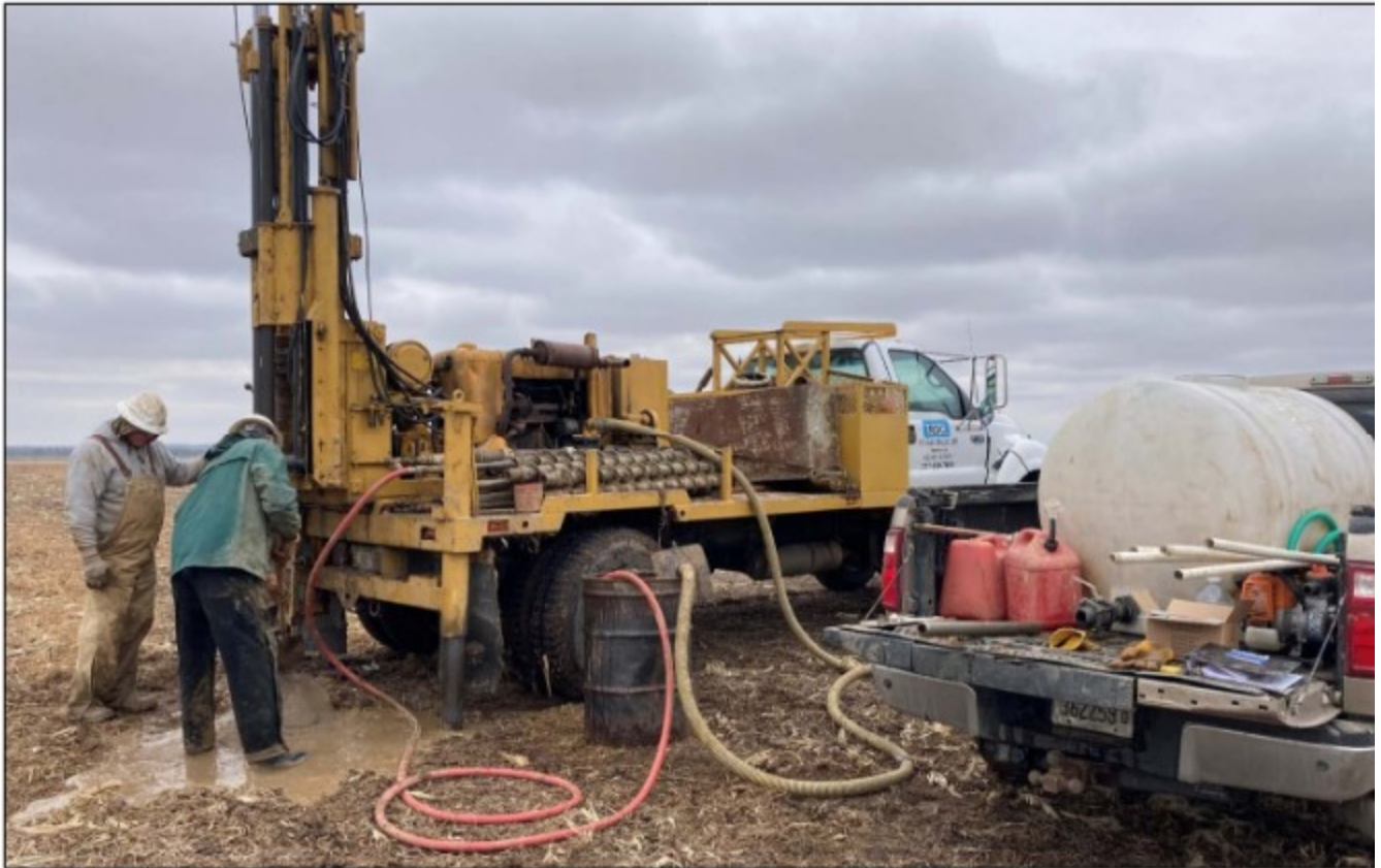
Truck-mounted rotary drilling rig
