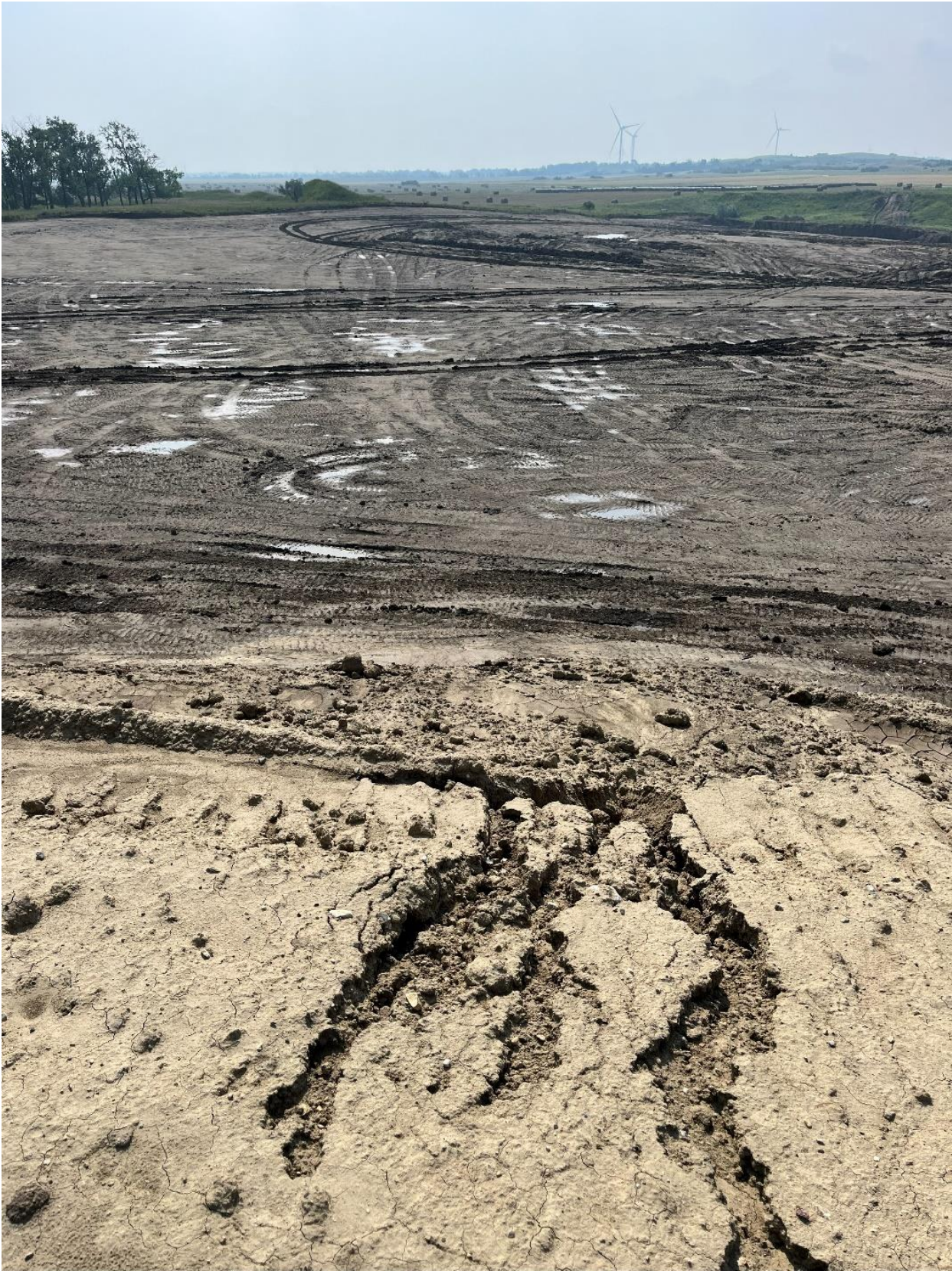
Figure 5: Dealing with muddy conditions was a continuous problem during active construction.
