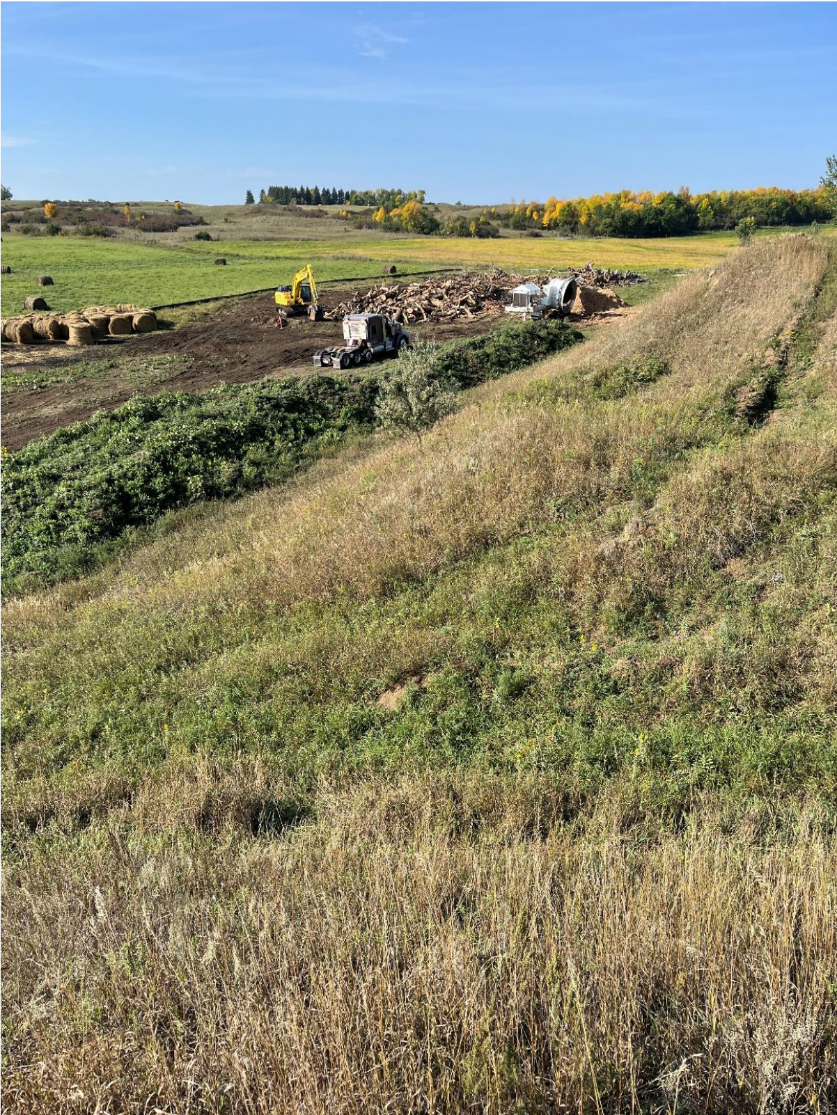
Figure 6: Over 600 trees were felled, shredded, and incorporated into the respread soil.
