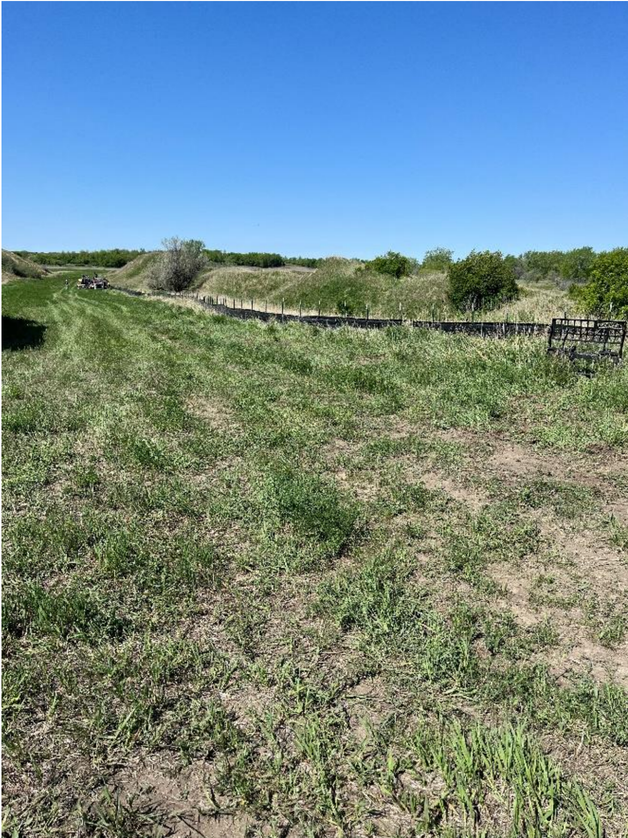
Figure 3: Over 3,800 feet of silt fence was installed to control sediment.
