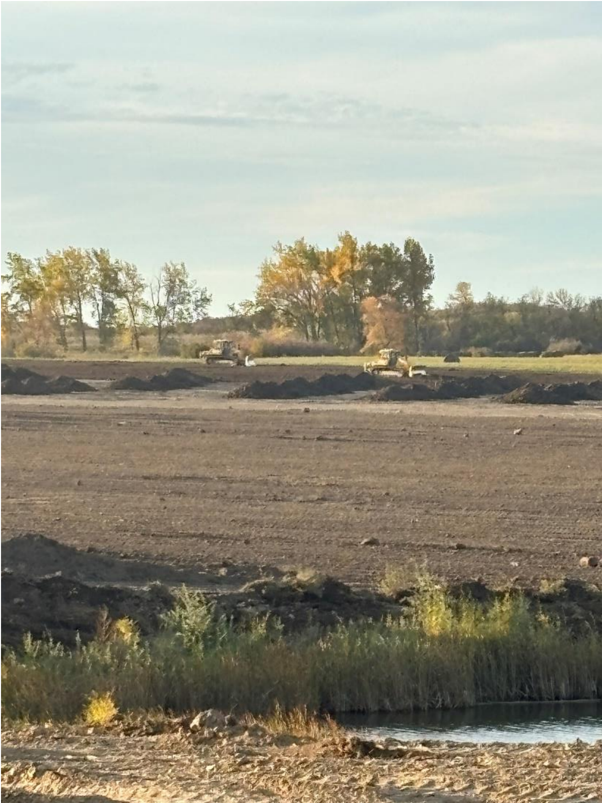
Figure 7: Dozers are respreading topsoil.
