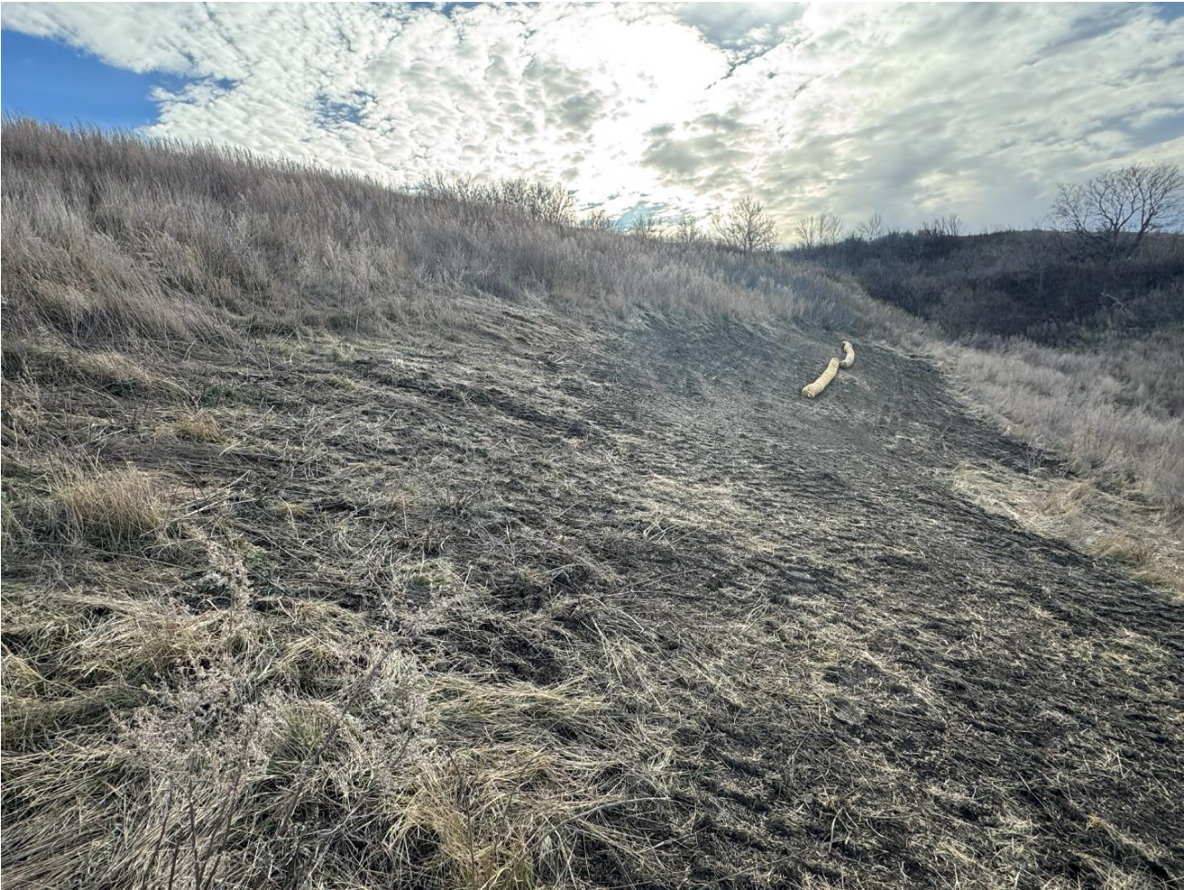
Figure 13: Repaired slope stability area after completion.
