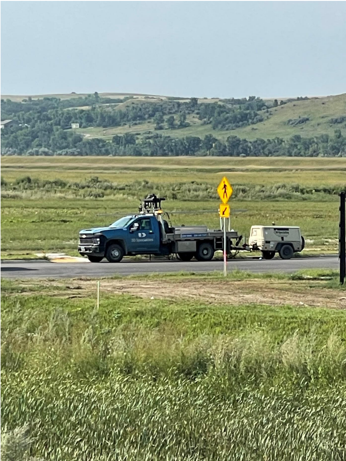
Photo 1: Dakota Fence at the location of installation with North crosswalk sign already installed.
